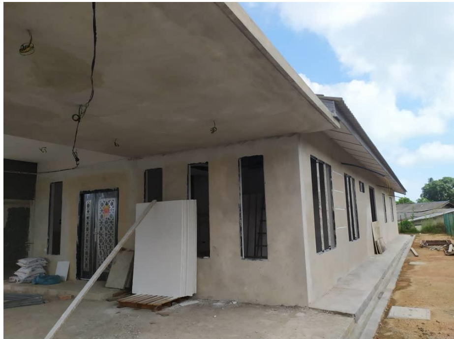
Figure 3.4 : Front view (right side) of the project at 70% progress.
