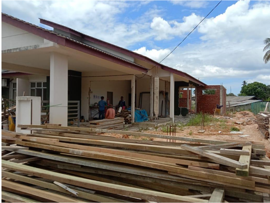
Figure 3.3 : Front view (right side) of the project at 10% progress.
