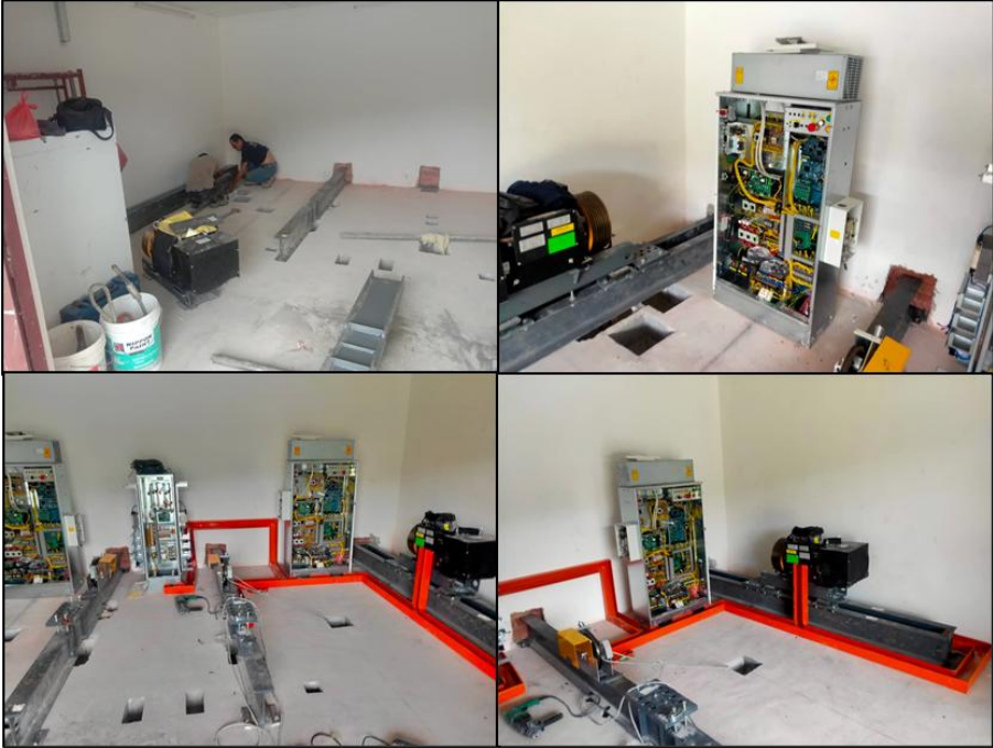
Figure 9: The installation of Traction Geared Elevator is currently underway
