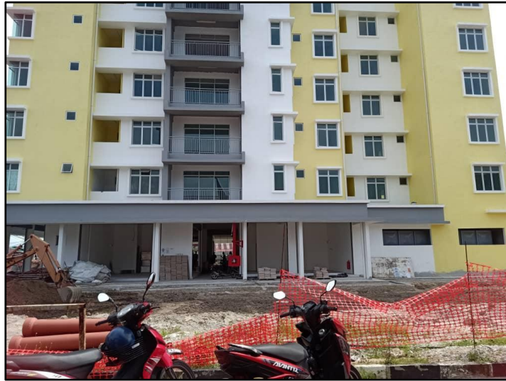
Figure 5: Conditions around the project site
