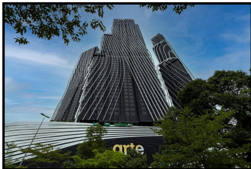
Figure 3.1.4 (a) : Front view of Arte Mont Kiara
