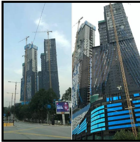
Figure 3.2: Building Construction of Arte Mont Kiara
