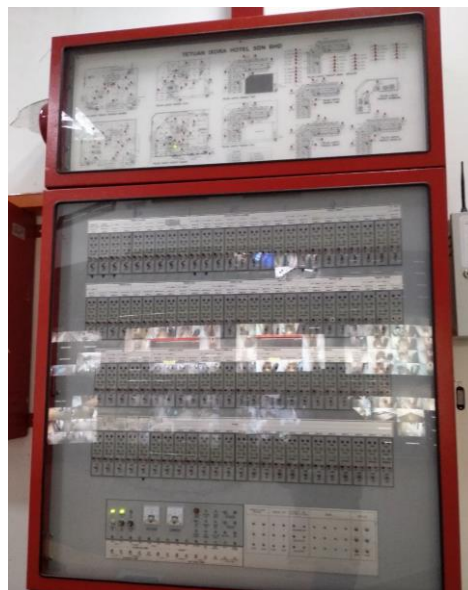
Figure 3.17: Fire alarms detectors and escape plan
