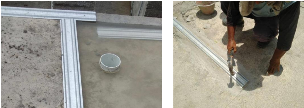
Figure 6: Installation of bottom track
