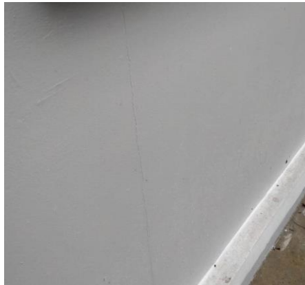
Figure 28: Crack at the joint
