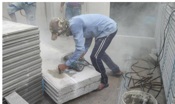
Figure 9: Cutting the panel wall
