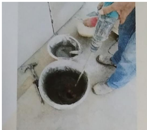
Figure 7: Applying bonding adhesive SIKA cream
