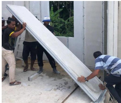
Figure 8: Installation of IBS lightweight panel wall
