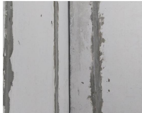
Figure 13: Applying hybrid mesh and skim coating to the panel wall.
