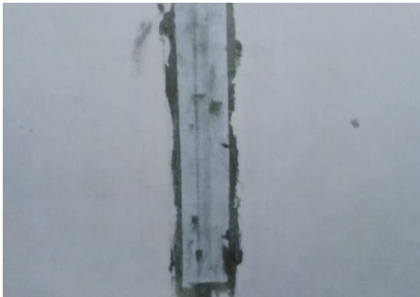
Figure 13: Applying hybrid mesh and skim coating to the panel wall.
