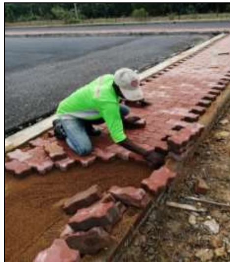
Figure 3.3: The Installation of Red Unipave at Lawn Bowl
