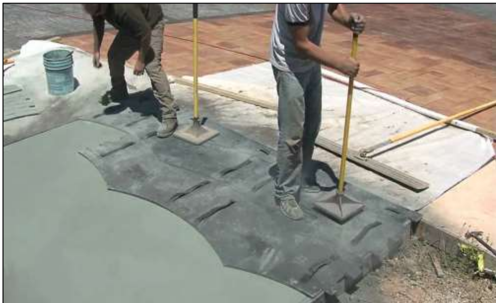
Figure 3.6: The Installation of Concrete Imprint at Driveway of Indoor Stadium
