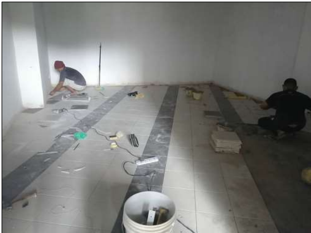
Figure 3.5: The Installation of Ceramic Floor Tiles at Surau of Indoor Stadium
