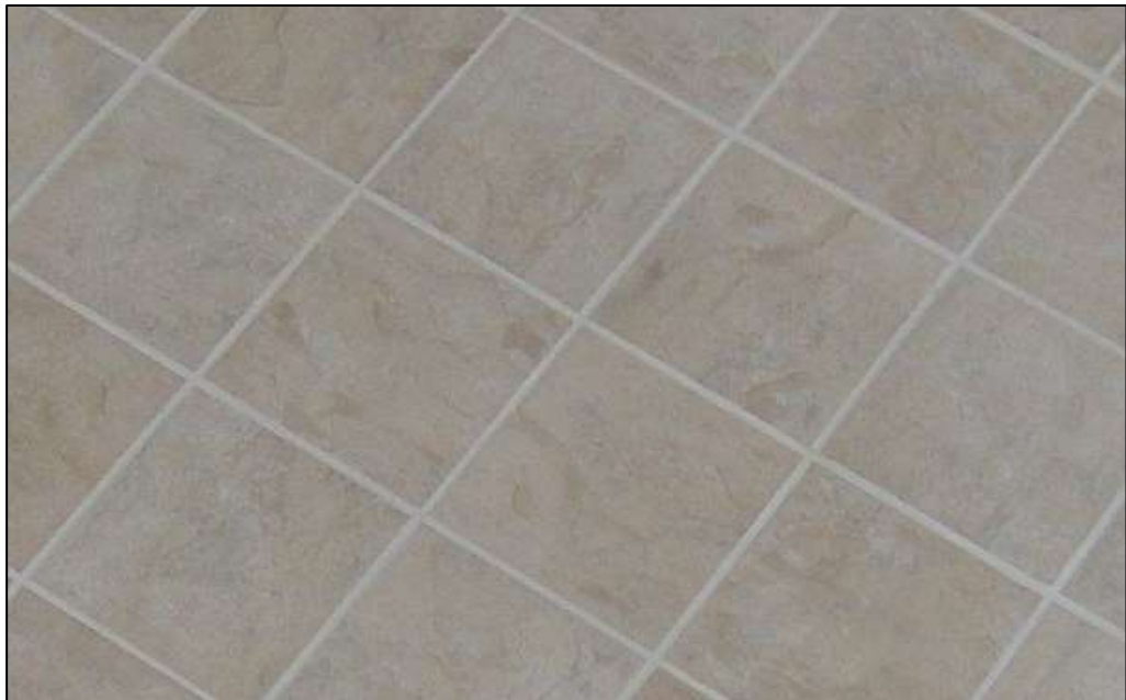
Figure 3.2: The Installation of Non-Slip Homogeneous Tiles at Kompleks Sukan Hulu Terengganu.
