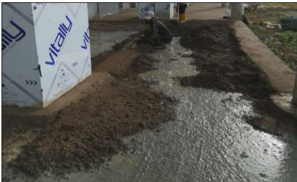
Figure 3.1: The Installation of Cement Screed at Corridor of Indoor Stadium
