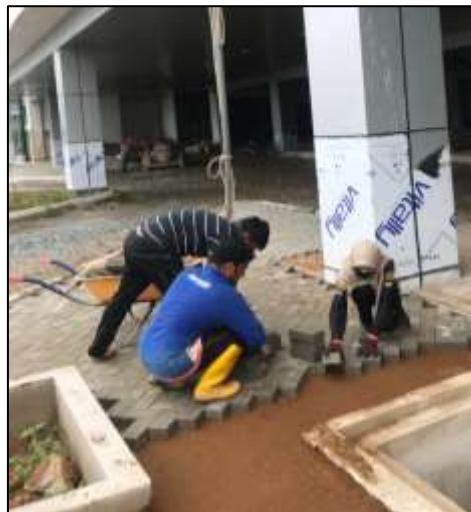
Figure 3.4: The Installation of Grey Flexipave at Indoor Stadium
