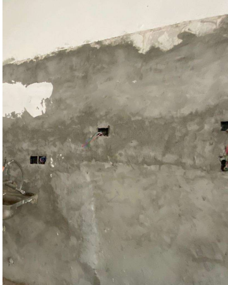
Figure 7: Plastering work at the kitchen
