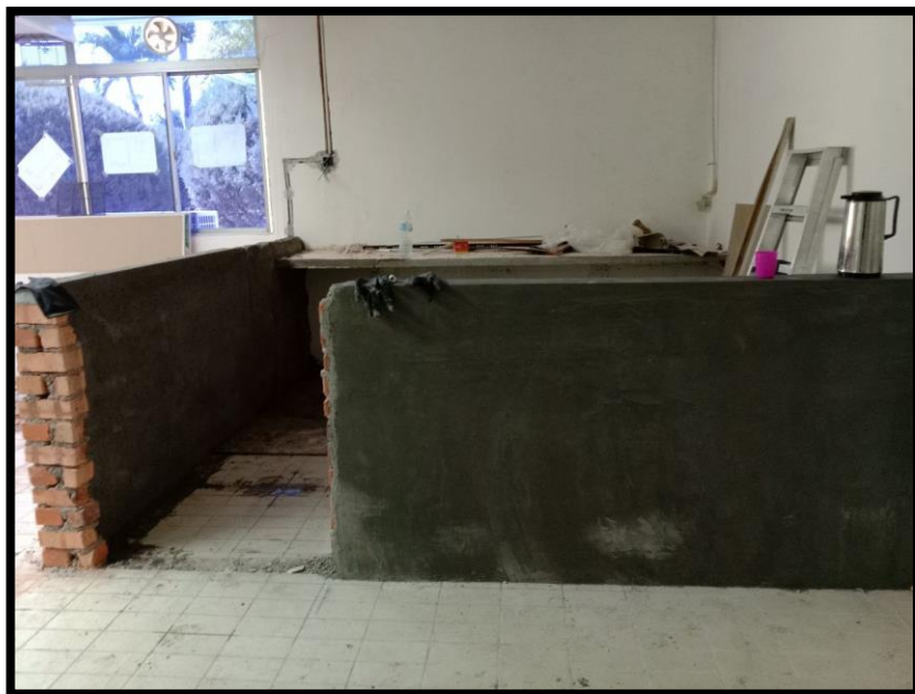
Figure 10:Brickwall for office room
