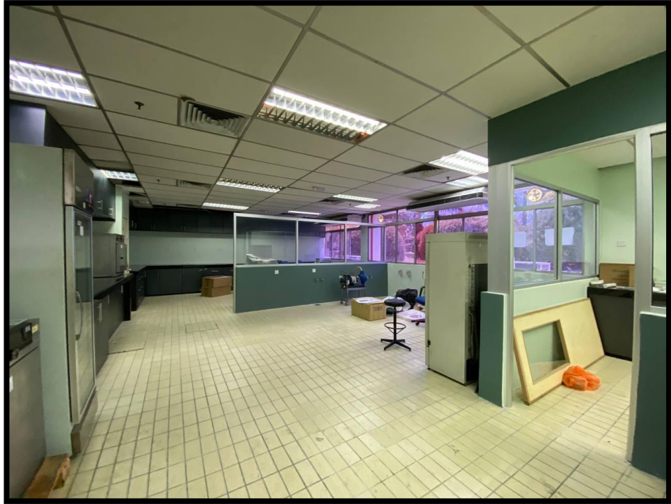
Figure 11: Overall view of the renovated lab room
