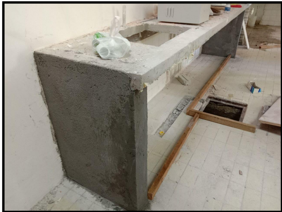
Figure 6: Concrete bench in Progress
