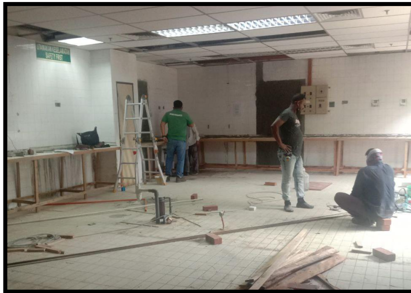
Figure 4: Workers doing work preparation
