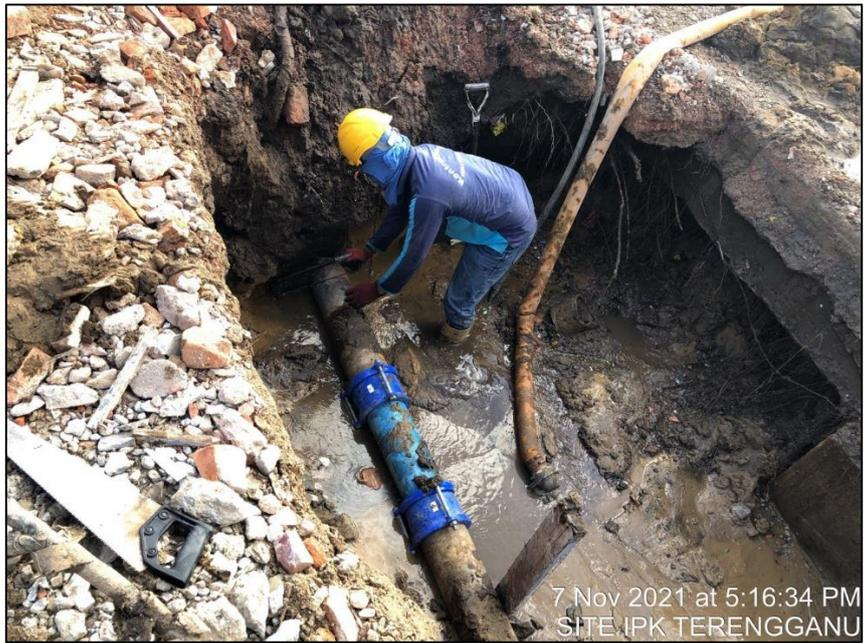
Picture 27: Water Reticulation Pipe Reparation Work
