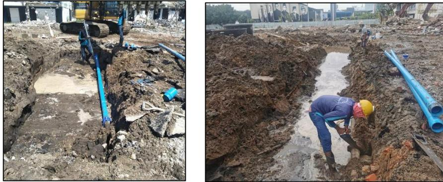
Picture 21: Water Reticulation Leakage
