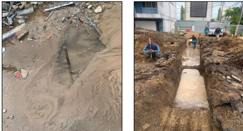
Picture 22: Water Reticulation Repair Work
