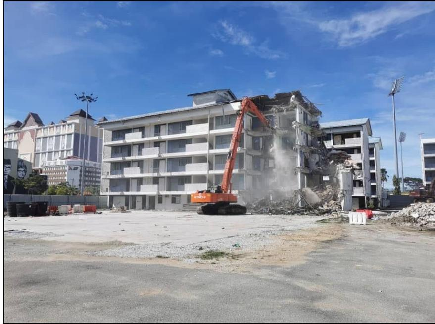
Picture 28: Long-reach Excavator Demolition
