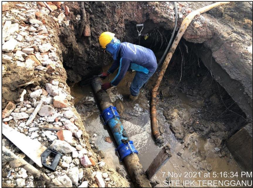
Picture 27: Water Reticulation Pipe Reparation Work
