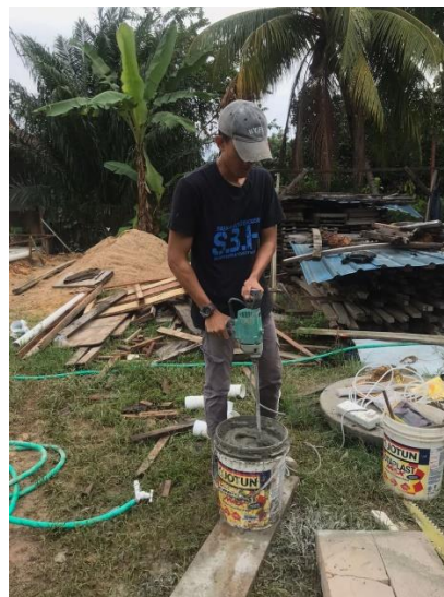
Figure 3. 19 Mixing thin-bed mortar
