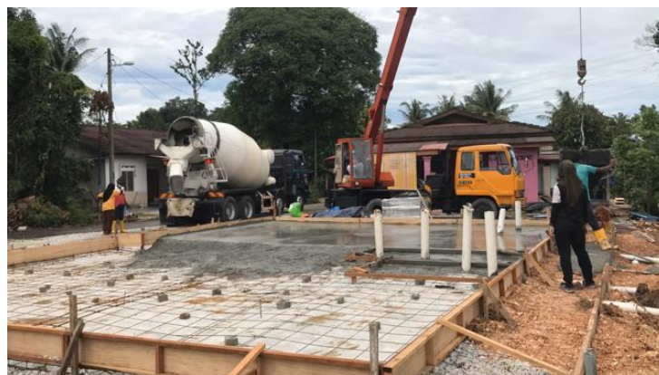
Figure 3. 11 Pouring concrete into the foundation
