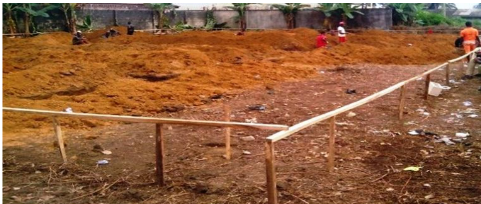
Figure 3. 5 Setting out
