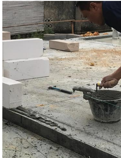
Figure 3. 16 Place mortar
