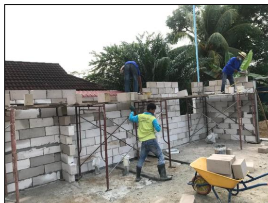
Figure 3. 23 Binding lightweight block
