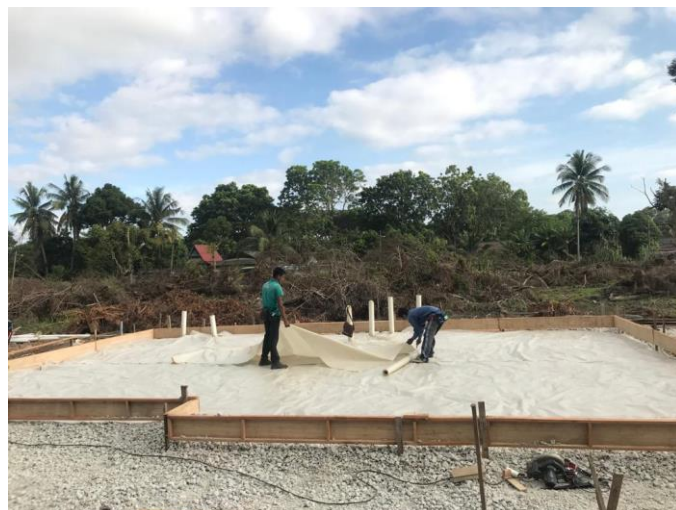
Figure 3. 9 Install P.E. Sheet
