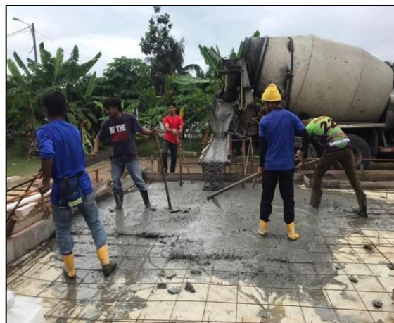
Figure 3. 36 Concreting the raft foundation
