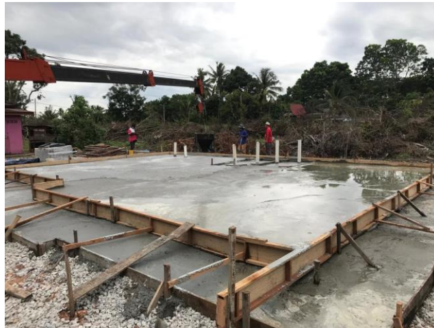
Figure 3. 13 Raft foundation
