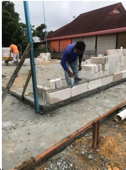
Figure 3. 20 Continuous levelling course
