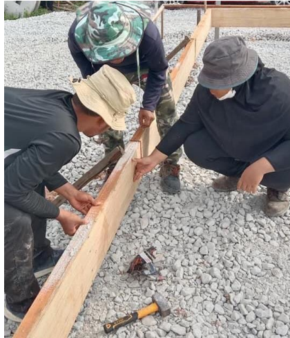
Figure 3. 8 Install formwork
