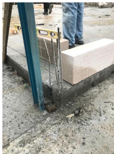
Figure 3. 17 Set the first corner block
