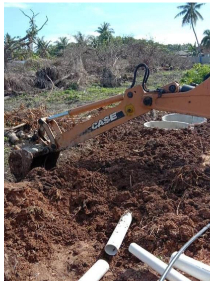
Figure 3. 34 Installing the septic tank
