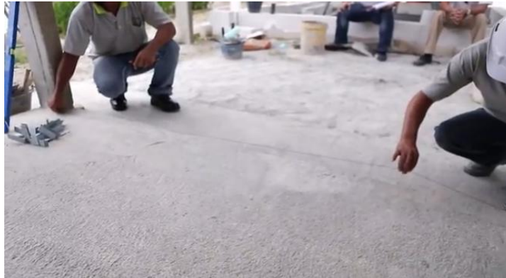
Figure 3. 14 Lay out wall line
