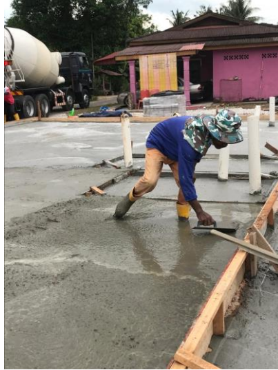
Figure 3. 12 Levelled the concrete
