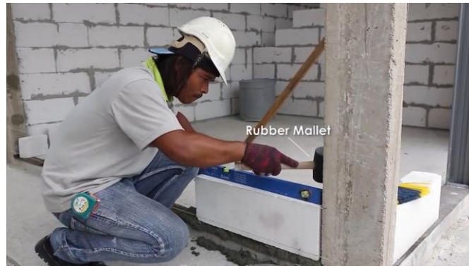
Figure 3. 18 Tapping down with rubber mallet
