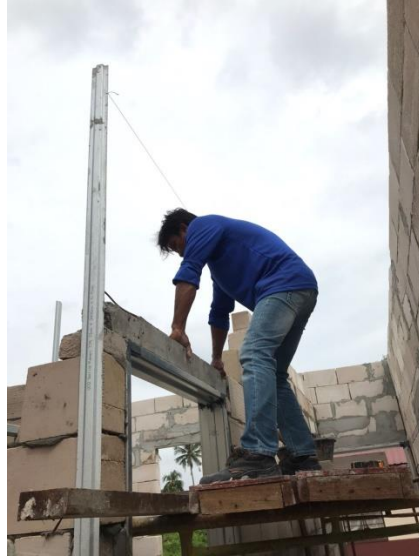
Figure 3. 21 Install lintel
