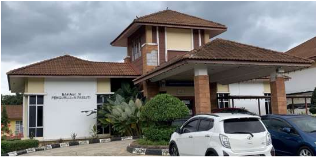
Figure 2.1: Front of Main Office
