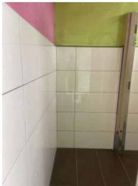
Figure 3.3: Homogeneous Tiles has been selected
