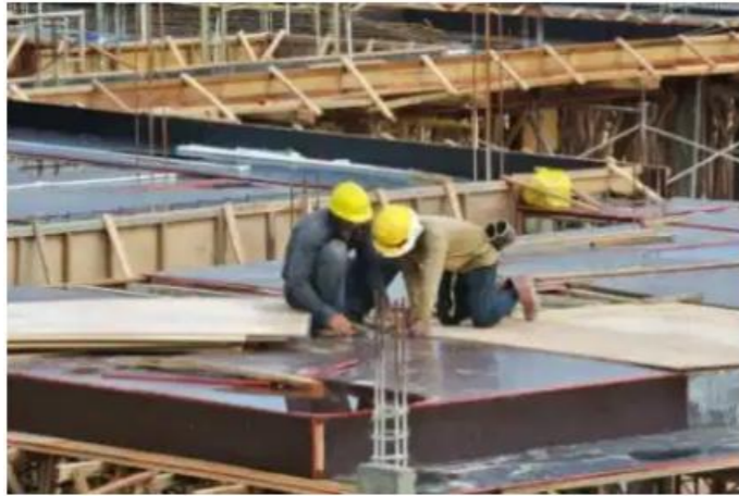
Image 2.0: Erection of Form work
