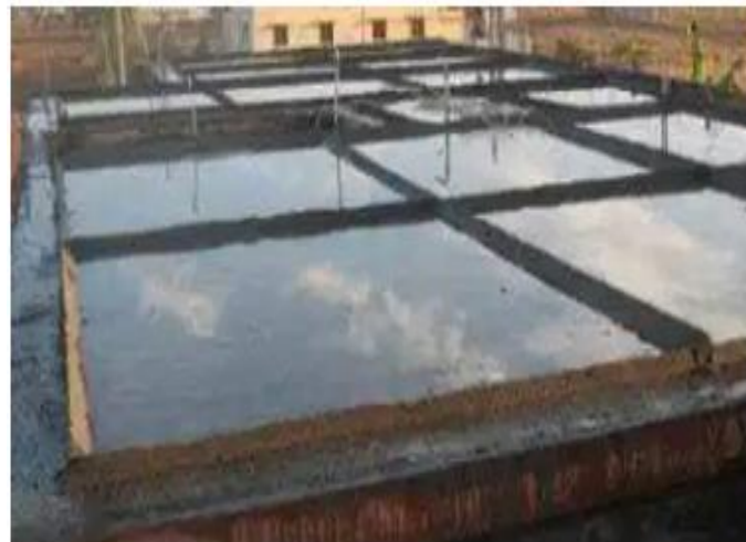
Image 2.3: Curing Concrete
