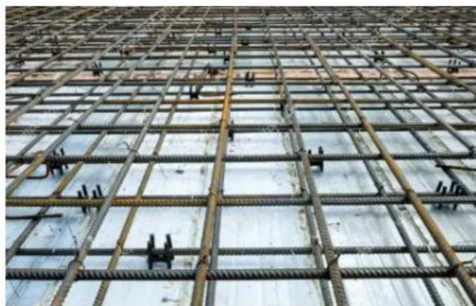
Image 2.1: Placement of Reinforcement
