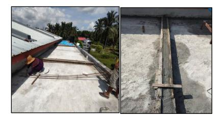
Photo 3:31 Process of create divider beam
