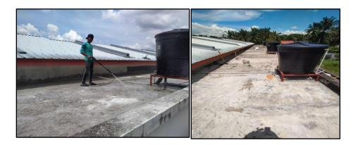
Photo 3:28 Process of claning flat roof
