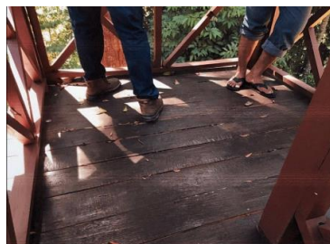
Figure 4.24: Floor Dormitory Before Maintenance
