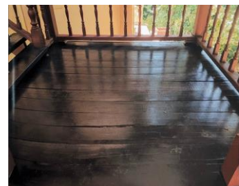
Figure 4.25: Floor Dormitory After Maintenance
