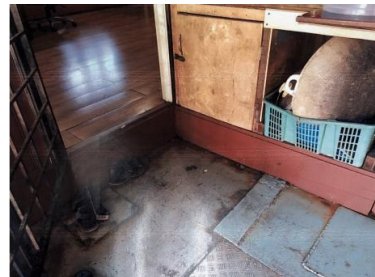
Figure 4.6: Office Floor Before Maintenance
