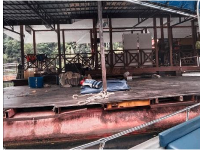
Figure 4.1: Kayak Storage Store Before Maintenance
