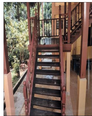
Figure 4.23: Railing After Maintenance
