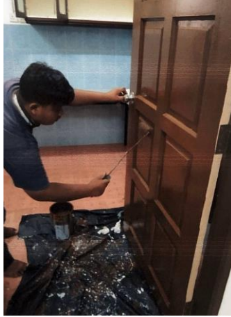
Figure 4.18: Door During Maintenance
