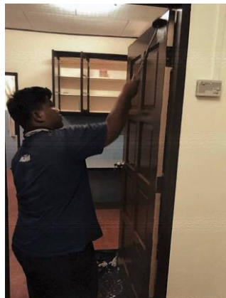
Figure 4.26: Door Dormitory During Maintenance
