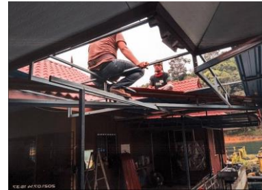
Figure 4.9: Awning During Maintenance
