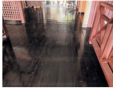
Figure 4.7: Wooden Floor on Jetty Lobby Maintenance
