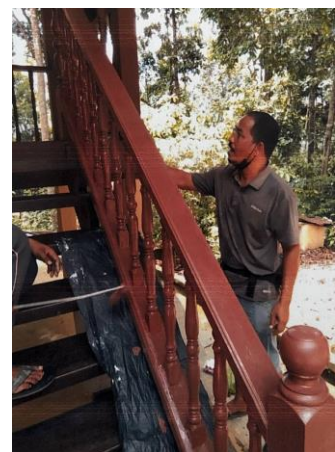
Figure 4.21: Railing During Maintenance
