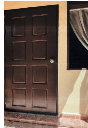
Figure 4.27: Door Dormitory After Maintenance
