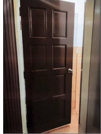
Figure 4.19: Door After Maintenance
