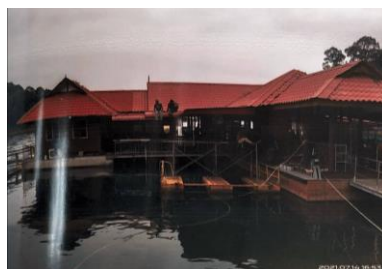
Figure 4.10: Awning After Maintenance
