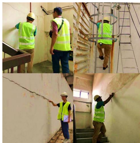
Figure 3.2.1 Building Surveyor make an inspection at the building.
