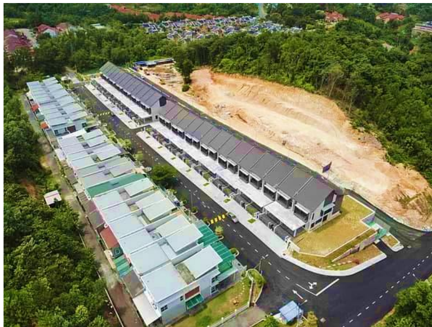
Figure 5.1.1: No 25 until No 52, Residential Double Storey Terrace At Taman Keruing, Sg Merab, Kajang From
