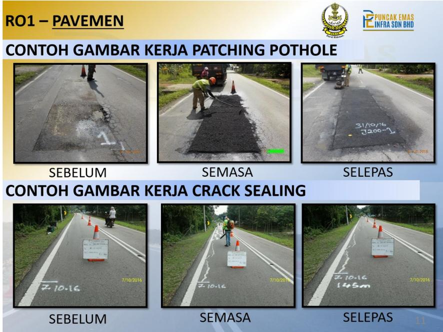
Figure 14: On-site work for patching pothole and crack sealing
