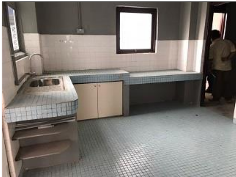
Figure19: Kitchen after repairing work
