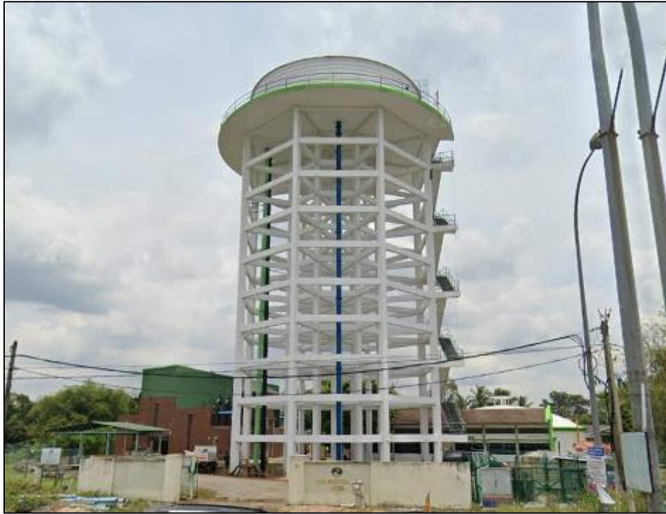
Figure7: Water tank tower
