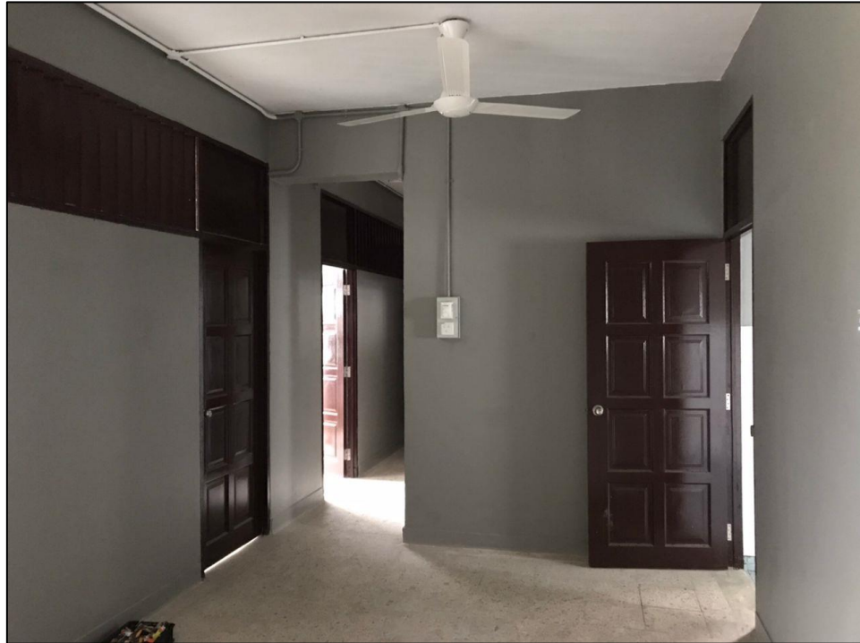
Figure20: Living room after repairing work
