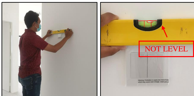
Figure 3.14: Spirit level is used on M&E outlets
