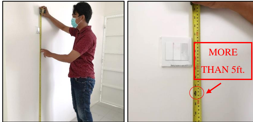
Figure 3.15: Steel measuring tape used to measure the height of M&E outlets
