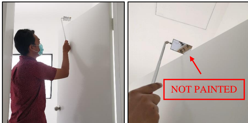
Figure 3.17: Angle mirror is used on the door
