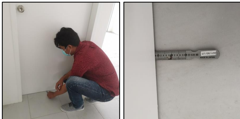
Figure 3.18: Steel wedge is used on the door
