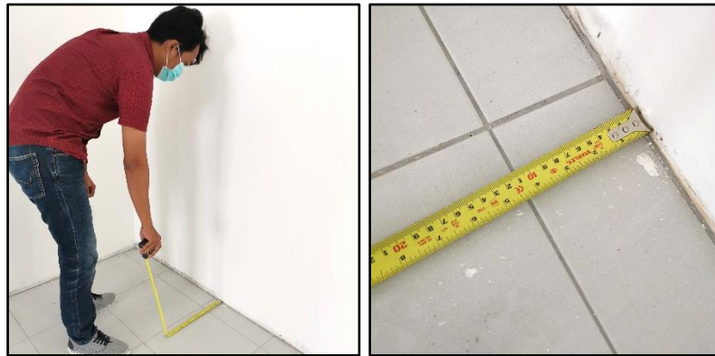
Figure 3.16: Steel measuring tape used to measure the uniformity of cut tiles
