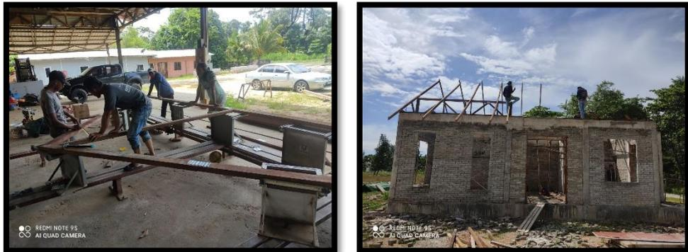
Figure 2 : *Installation of wooden IBS at the factory and construction site*
