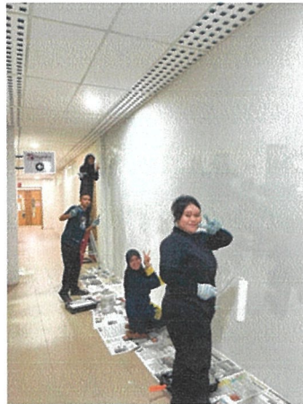
Painting Front Office Wall
