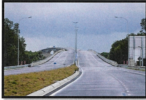
Figure 5.3.3.1 Sungai Pulai Bridge
