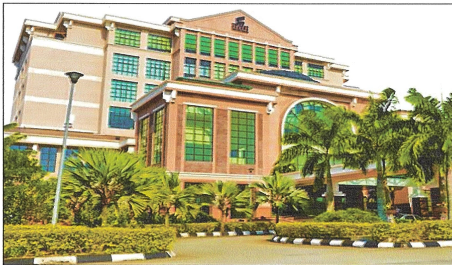
Figure 2.2 Building of UCYP's Office
