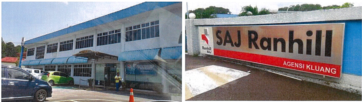
Figure 3: Ranhill SAJ Building
