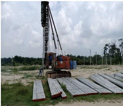
A machine that been use to penetrate the pile into the ground.
