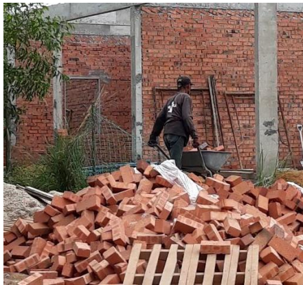
Figure 3.9: Lifting brick using wheelbarrow from stock pile
