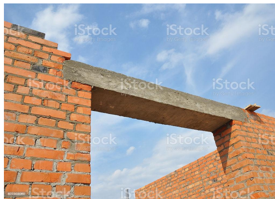
Figure 3.16: Lintels That Used As Load Support At the Top Of Opening Parts
