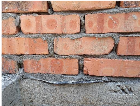
Figure 3.12: Install Damp Proof Course Under Between The Bricks
