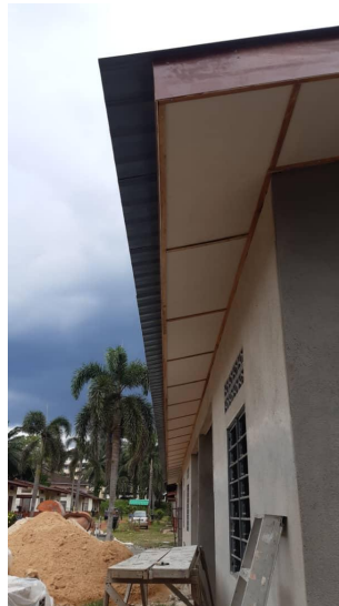
Figure 3.18: The wall after finish plastering process
