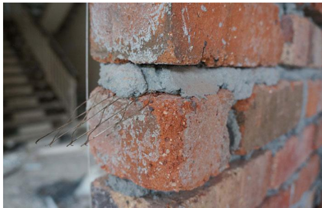
Figure 3.14: An exmet wire inside the layer of the brick wall
