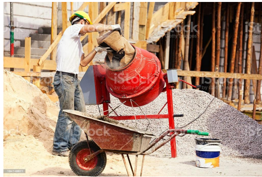
Figure 3.10: Mortar are mixed using the concrete mixer
