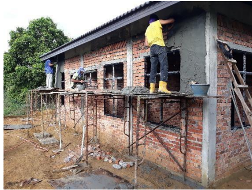
Figure 3.17: Plastering the top of wall for the finishes
