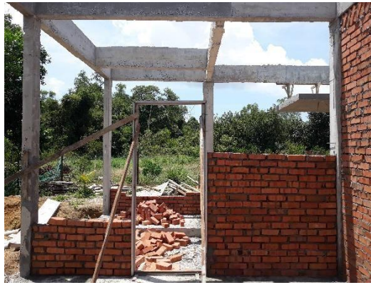
Figure 3.15: The view of door opening part of the wall
