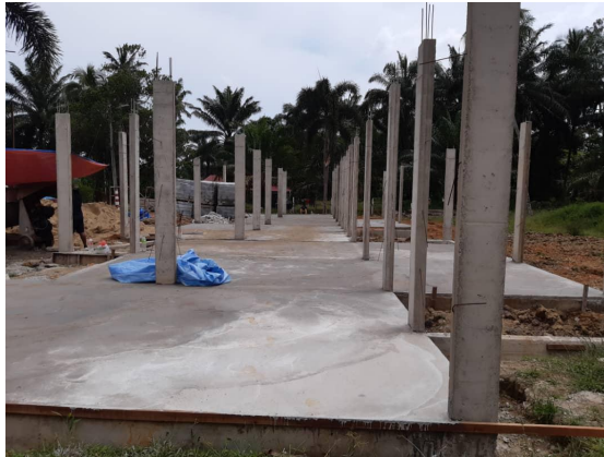
Figure 3.8: Floor that have been clean before brickwork process
