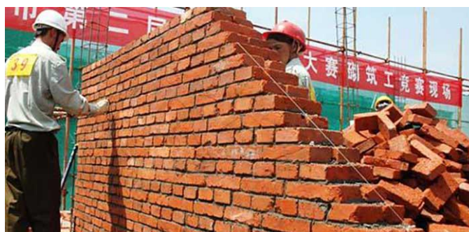
Figure 3.13: Brickwork the wall (Brick Wall) process
