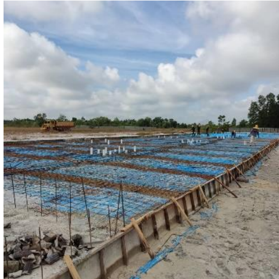
Figure 3.12: install the formwork and BRC for ground beam and footing
