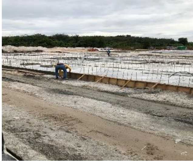
Figure 3.16: Remove formwork
