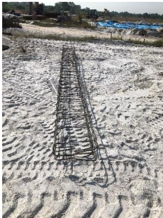
Figure 3.8: the Rebar for footing
