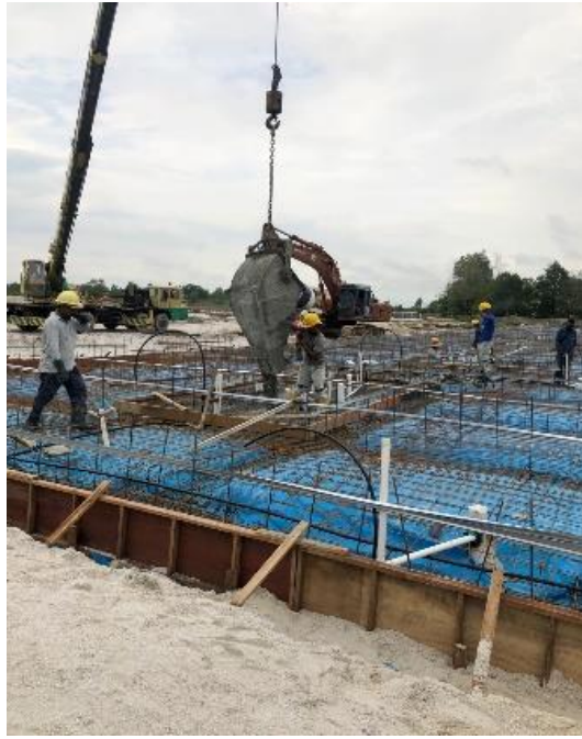
Figure 3.14: concrete work with crane
