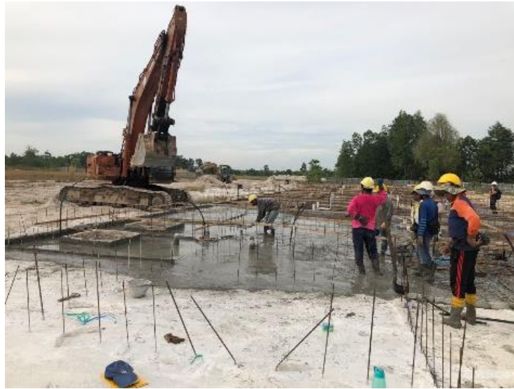
Figure 3.6: - the concrete work
