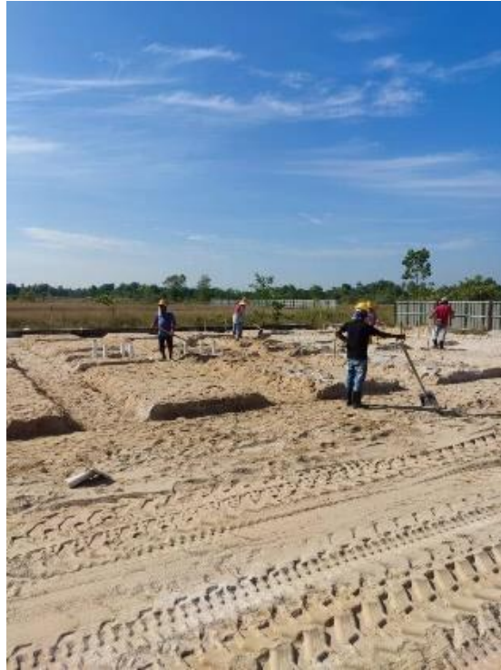
Figure 3.11.: excavate for slab
