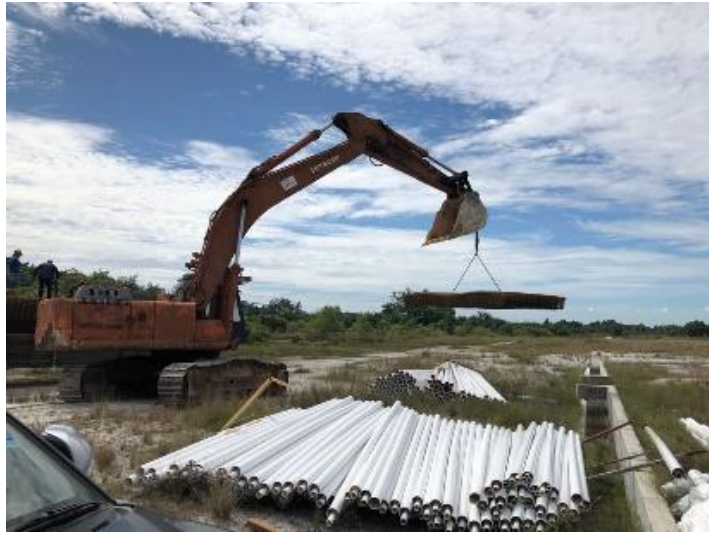
Figure 3.7: the steel reinforcement arrive at site
