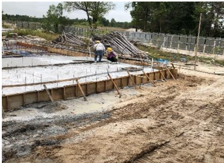
Figure 3.17: Remove Drop Formwork
