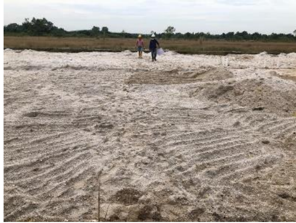
Figure 3.10: Setting Out in progress
