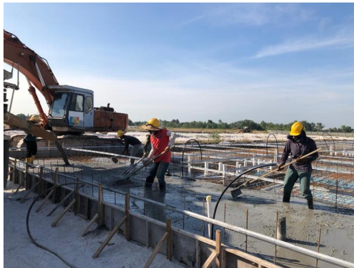
Figure 3.15: compact and flattening the concrete
