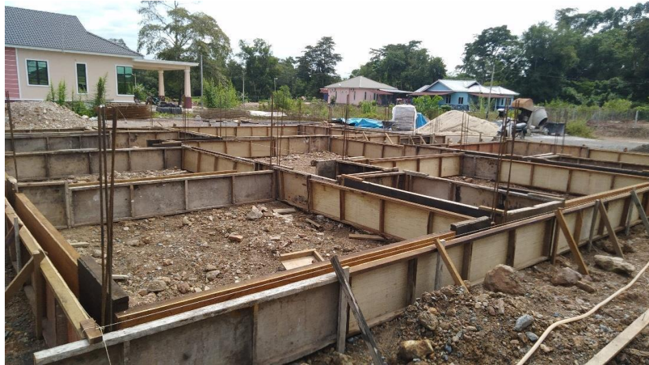
Figure 7.0: All the formwork that been installed.
