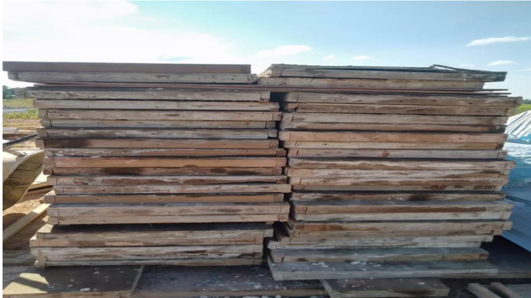
Figure 12.0: All the formworks has been gathered in one place
