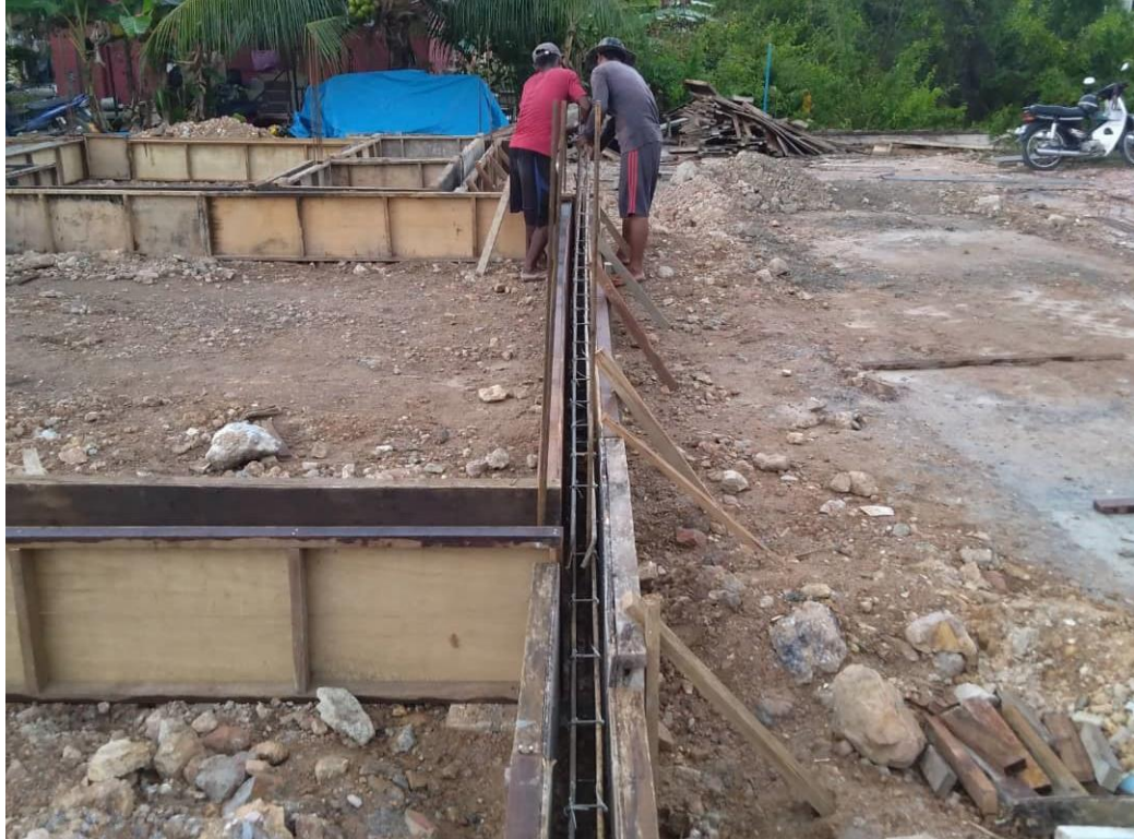
Figure 8.0: The labors were installing the reinforced bars into the formwork
