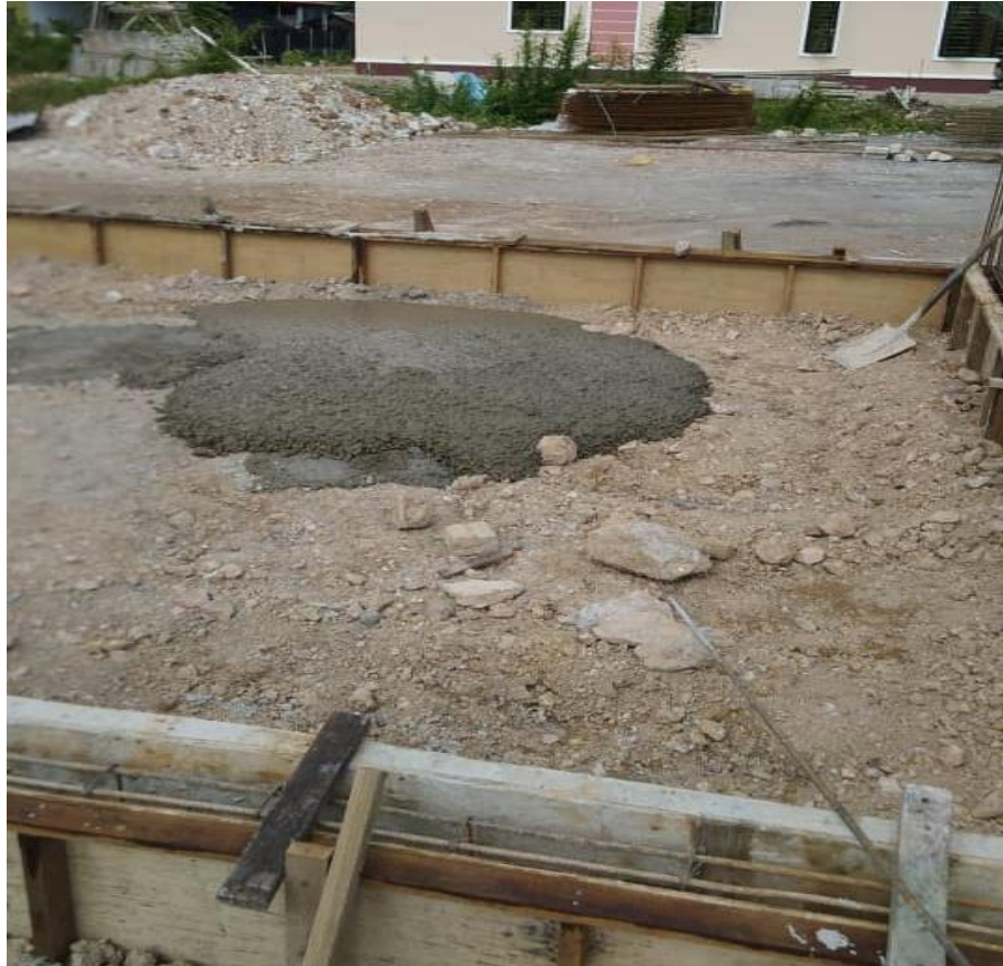
Figure 10.0: The balance of concrete that starts to harden that dumped by the truck.
