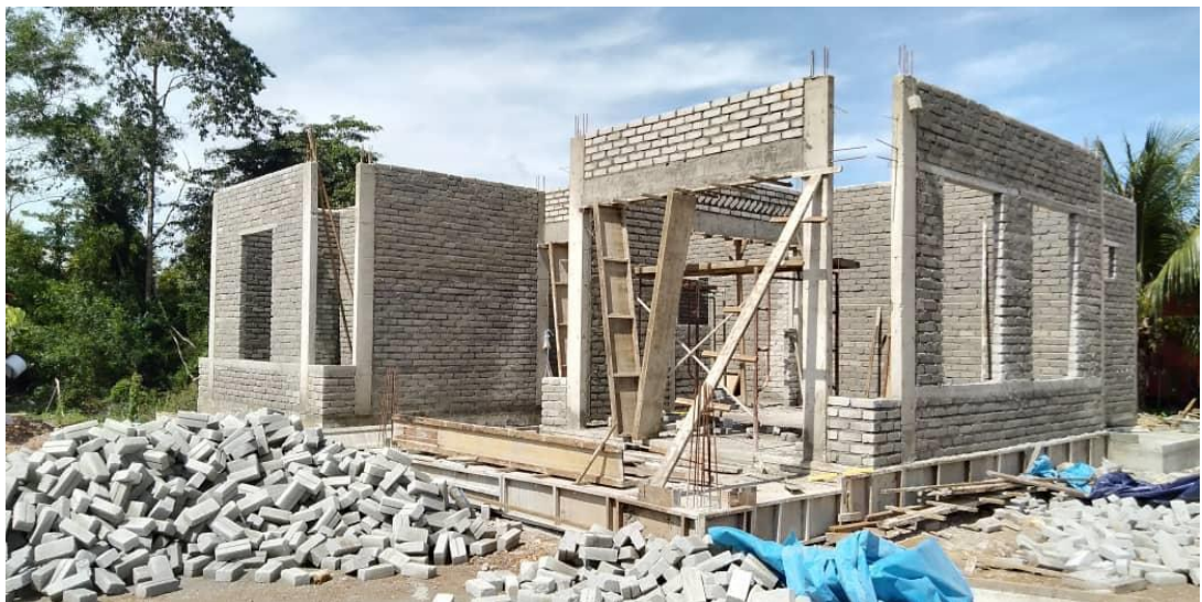
Figure 1.0: The actual building for this report in brickwork process
