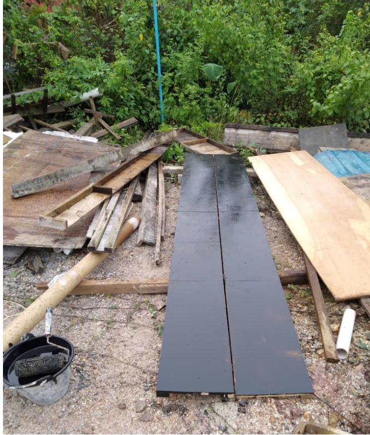
Figure 6.0: The beam formworks has been coated with black oil
