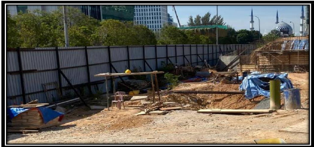
Figure 4: Silt Trap on Site
