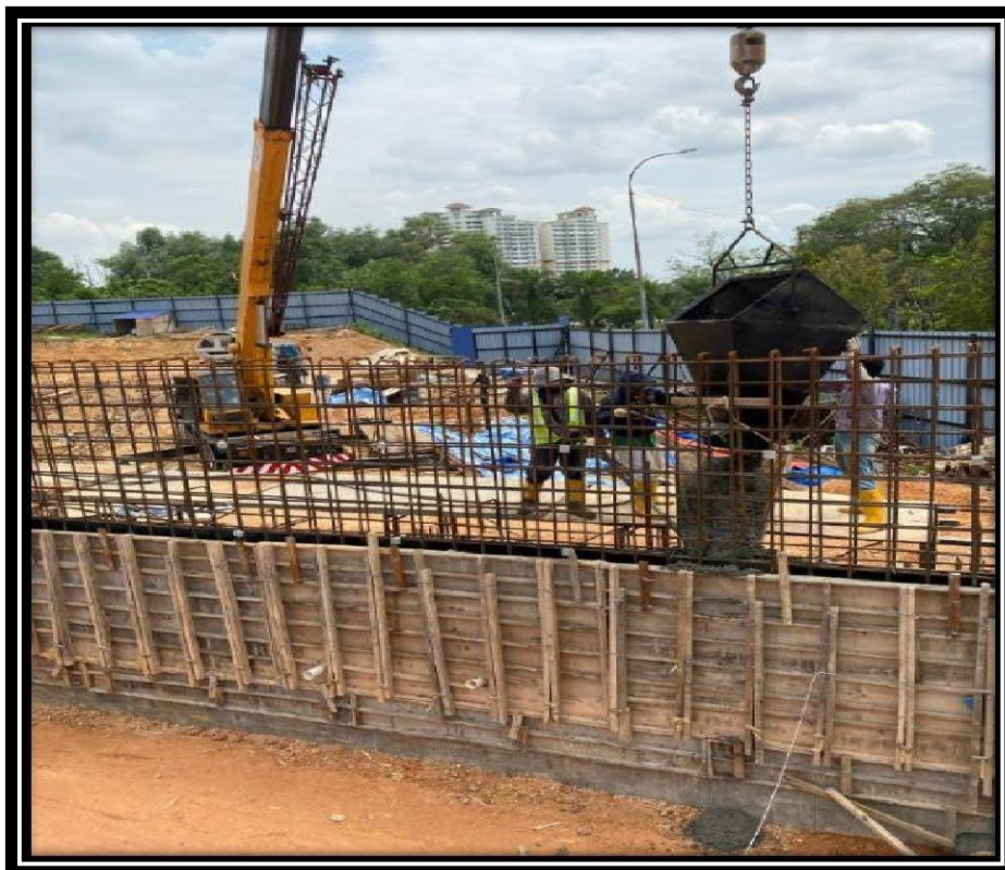
appendices 4:Shows concreting process for retaining wall
