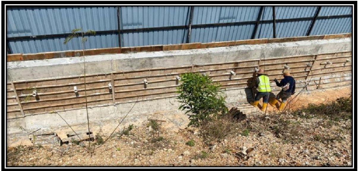
appendices 10:: Shows the dismantle of formwork after 7 days after concreting.
