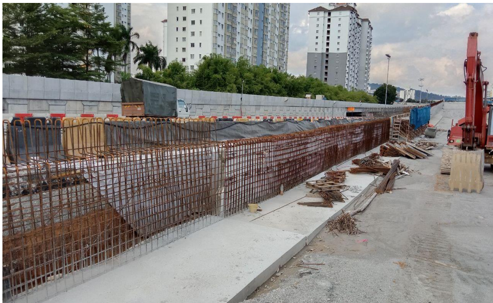
Figure 3.1.1: Levelling pad
