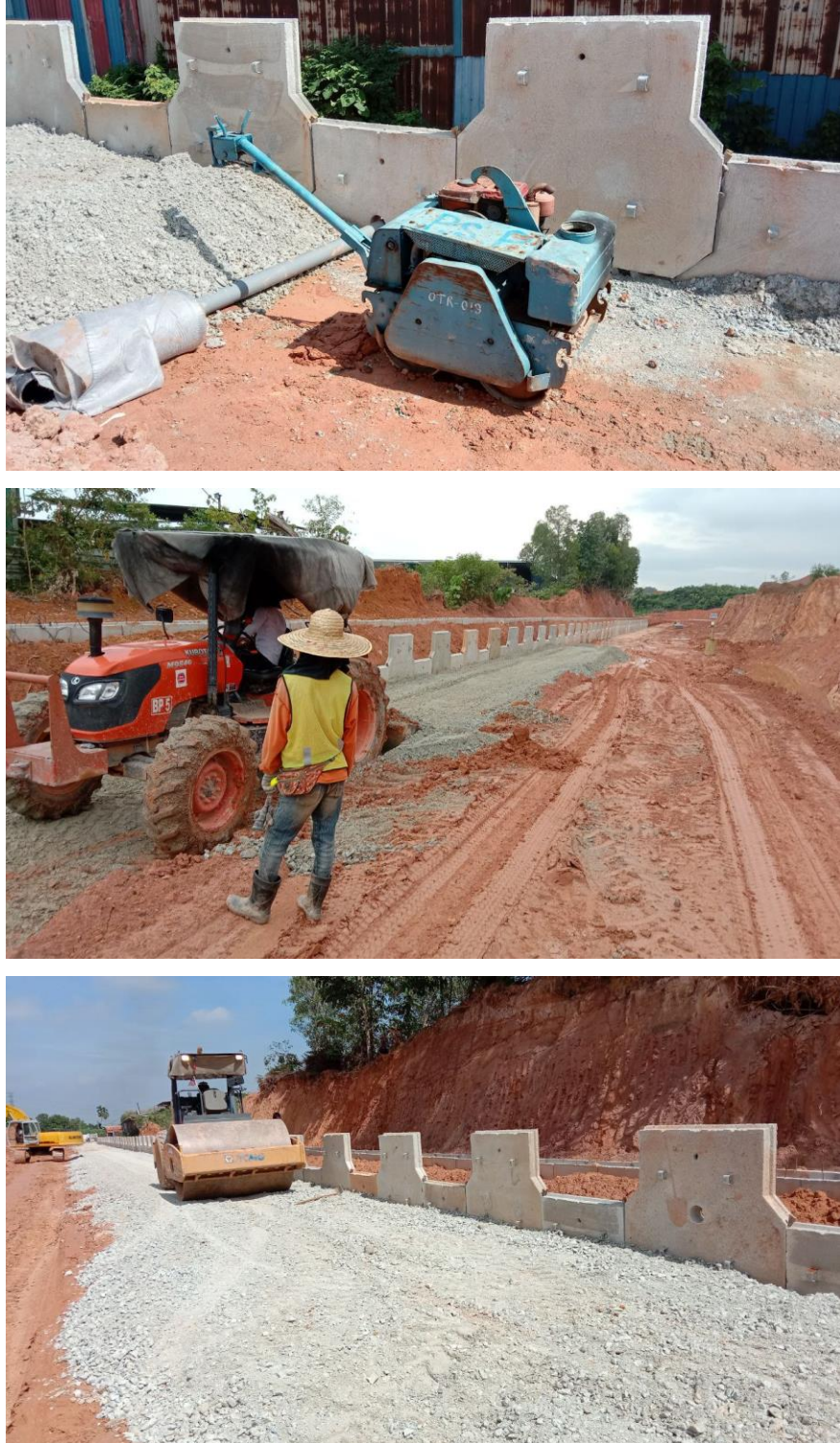
Figure 3.1.5.4: Compaction
