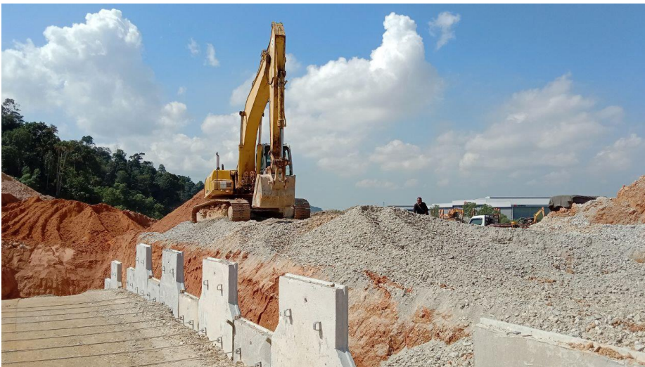
Figure 3.1.5.2: Backfill material
