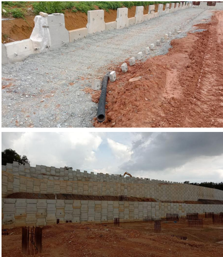
Figure 3.1.5.3: Installation panel wall
