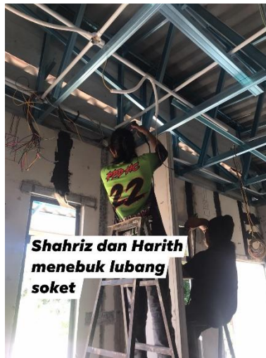
Figure 3.14: The holes were made using Hammer Drill
