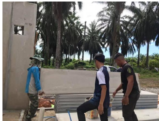
Figure 3.5: Precast Concrete Wall came in bundle.
