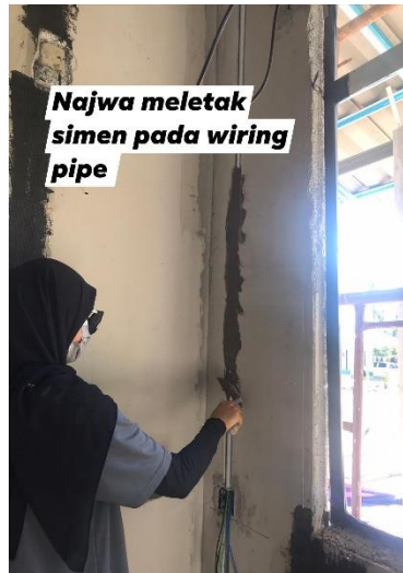
Figure 3.15: Closing the holes using cement
