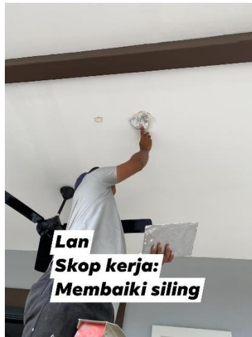
Figure 3.19: Worker covered the holes using Cornish Compound mixture
