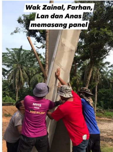
Figure 3.4: Installing Precast Concrete Wall required manpower
