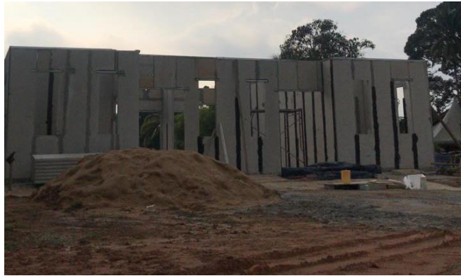
Figure 3.2: Project Bukit Tembakau at 40%
