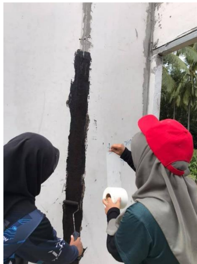
Figure 3.6: Applying fiber mesh net and UCO jointing compound.
