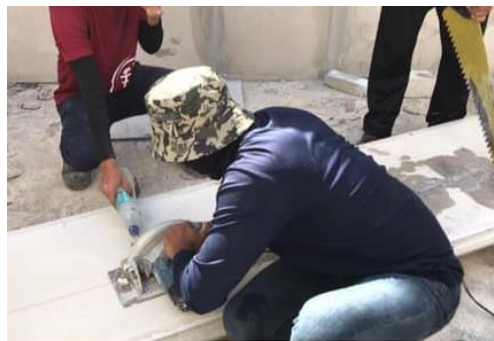
Figure 3.12: Worker cut the wall using Circular Saw
