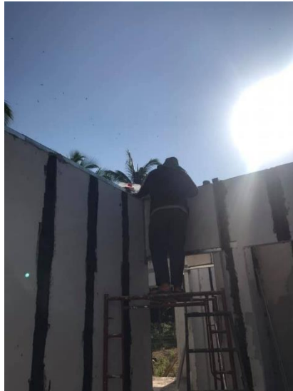
Figure 3.7: Applying top track to the wall
