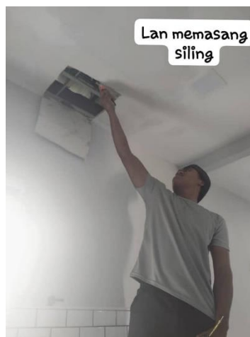
Figure 3.18: Worker replaced the damp ceiling with new ceiling board
