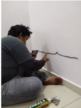
Figure 3.16: The cracks on the wall was closed using silicone
