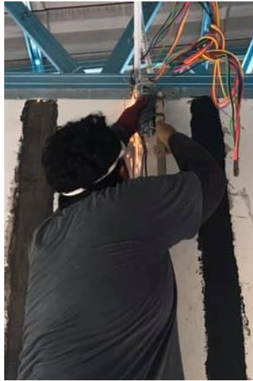
Figure 3.13: The walls were cut using Grinder
