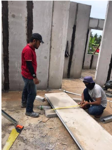
Figure 3.11: Worker measured the part to cut it
