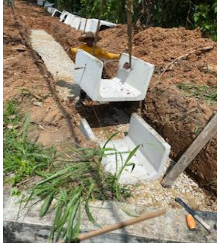
Figure 2.5 Install the drains
