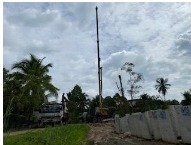
Figure 2.1 Lifting using crane
