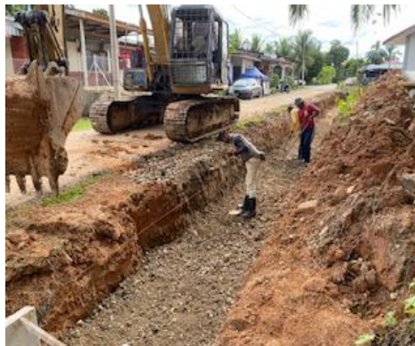
Figure 2.4 Spreading crusher-runs
