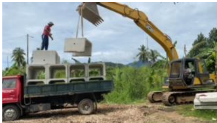
Figure 2.0 Lifting drain
