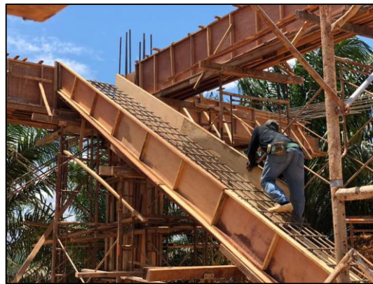
Figure 3.13: Sides formwork installation
