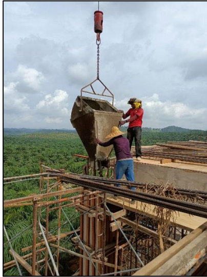
Figure 3.8: Column concrete pouring
