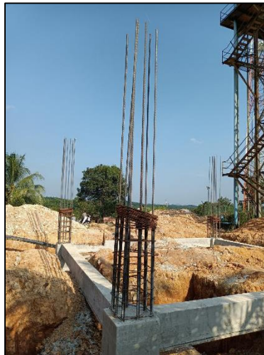
Figure 3.3: Column rebars
