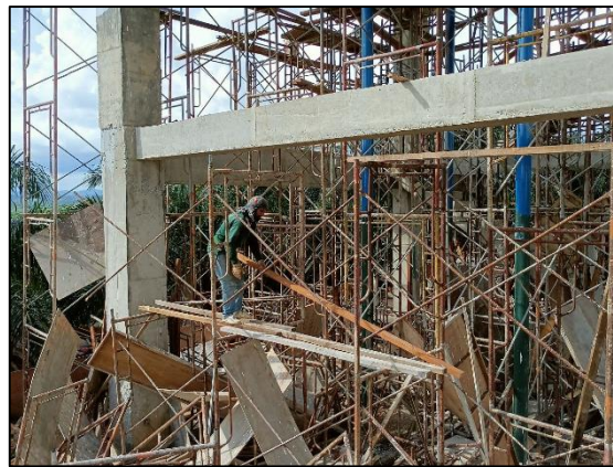
Figure 3.9: Column formwork dismantling process
