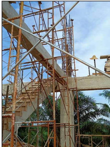
Figure 3.16: Staircase formworks dismantling process
