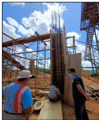
Figure 3.17: Steel checking progress
