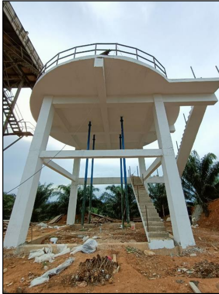
Figure 3.10: Column painting work
