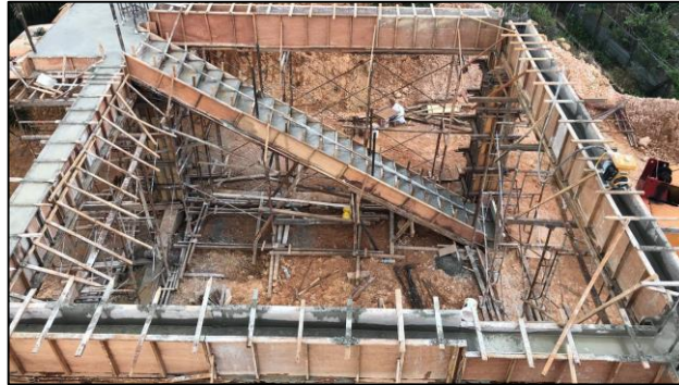
Figure 3.15: Concrete pouring to staircase
