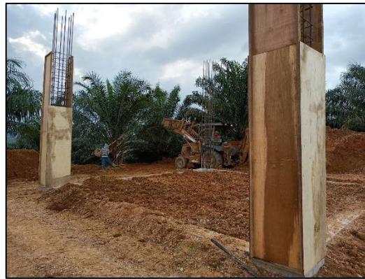
Figure 3.5: Column formworks
