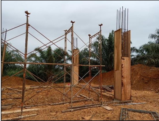
Figure 3.6: Scaffoldings installation
