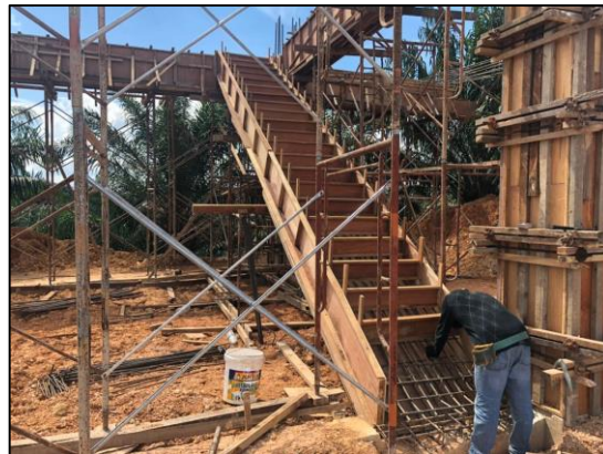
Figure 3.14: Riser formwork installation
