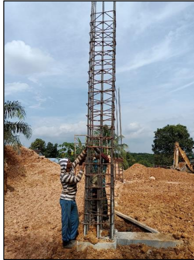
Figure 3.4: Column stirrups
