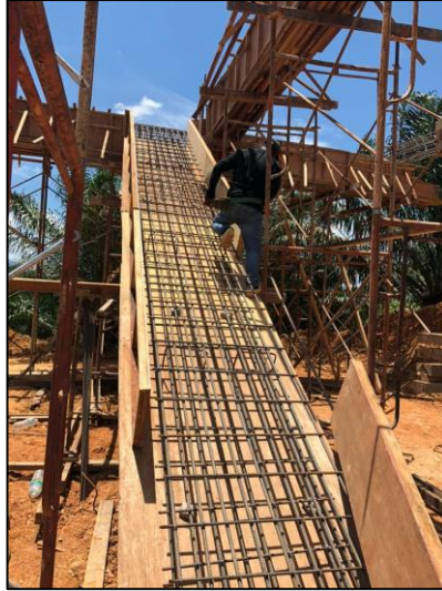
Figure 3.12: Rebar installation to staircase
