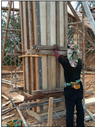
Figure 3.7: Column shutters installation
