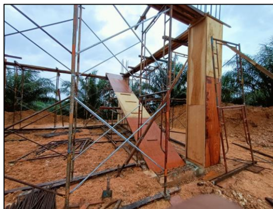
Figure 3.11: Formwork installation for soffit
