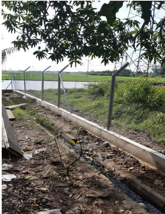
Figure 3.8.2: Condition of the fences kerb after construction
