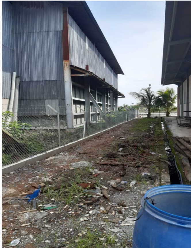
Figure 3.8.1: Fences condition after construction works
