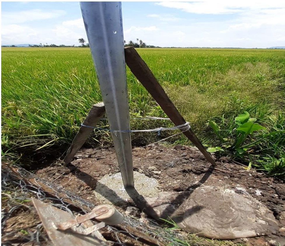
Figure 3.4.3: Positioned steel post after pouring a concrete
