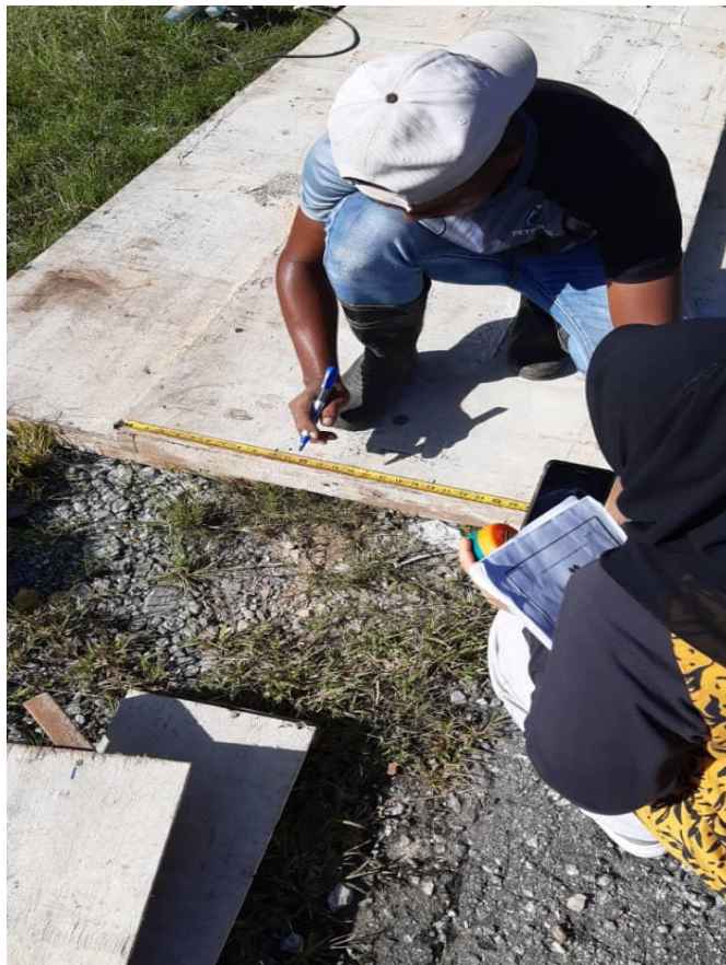
Figure 3.6.1: Formwork preparation
