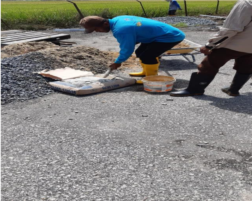
Figure 3.4.1: Workers prepared the cement mix for steel post installation
