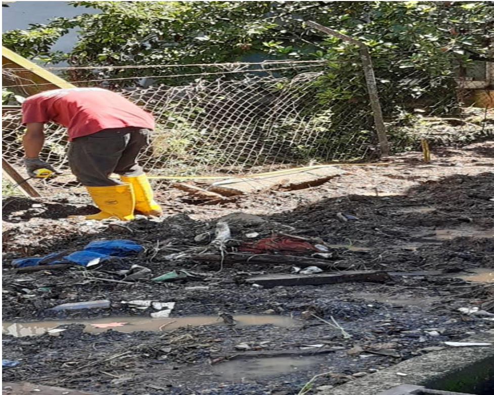
Figure 3.4.2: Placing peg and dig a 3 feet holes
