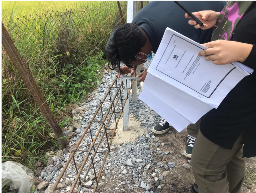
Figure 3.5.1: inspection of the bar and links for the fence slab
