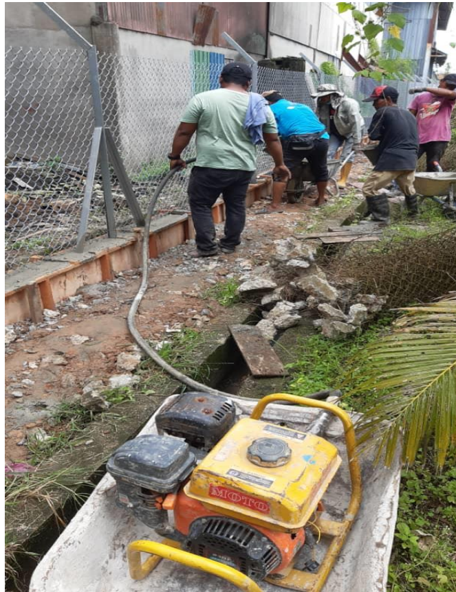
Figure 3.7.5: construction workers using concrete vibrator
