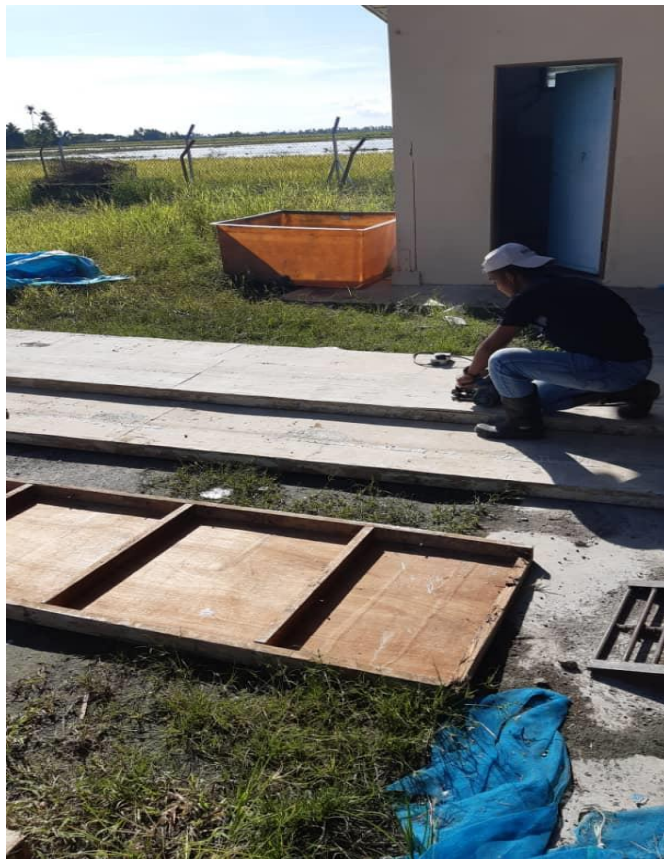
Figure 3.6.2: Formwork cutting
