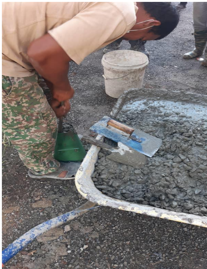
Figure 3.7.1: Slump test done by workers
