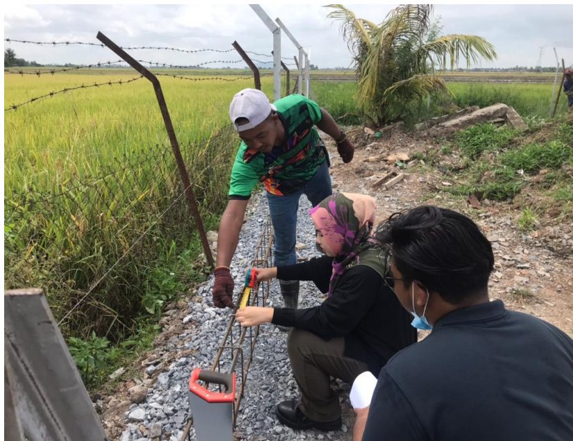
Figure 3.5.1: inspection of the bar and links for the fence slab
