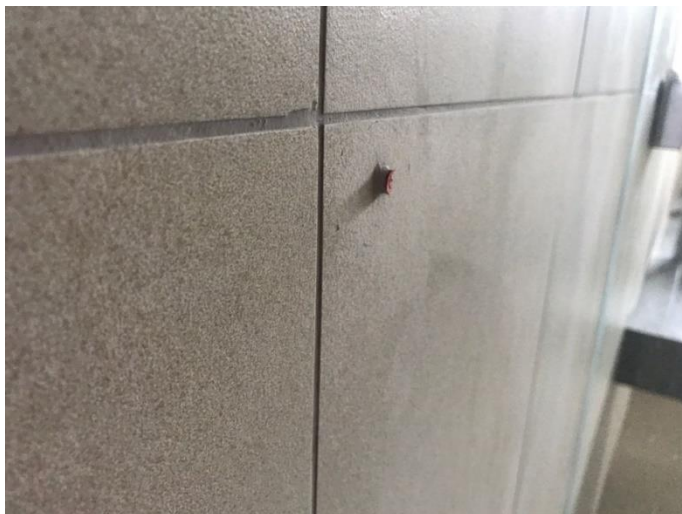
Figure 3.19: The Finished Work.
