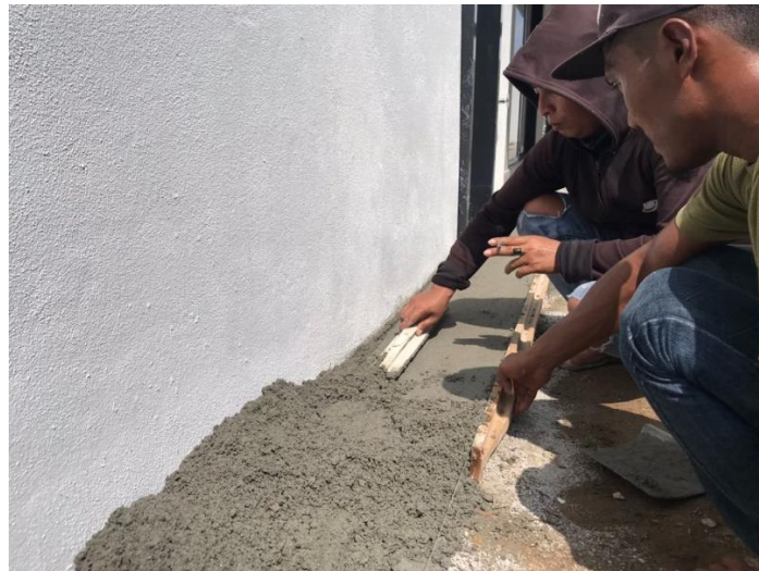
Figure 3.20: Progress of Rectification Works.
