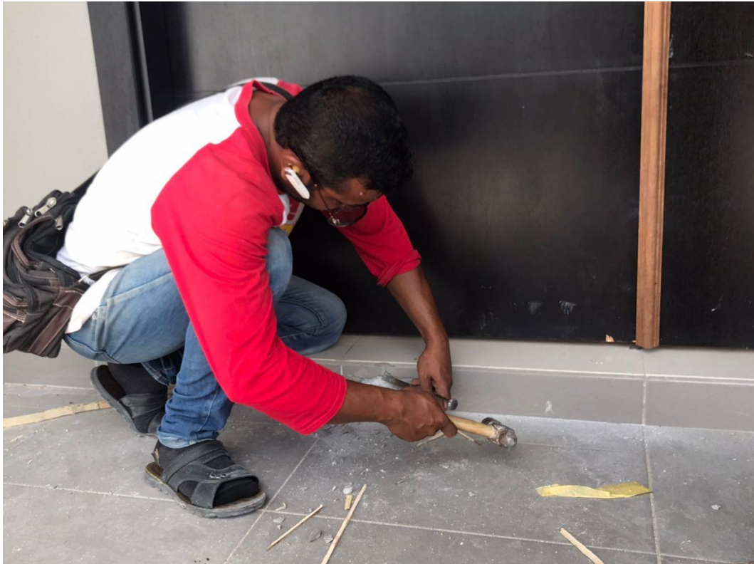
Figure 3.4: The Tiler Do The Rectification Works.
