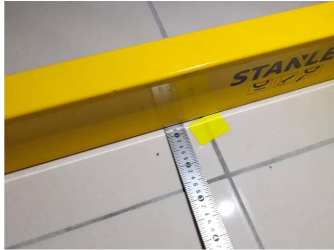
Figure 3.17: Checking the Tolerance with Spirit Level.
