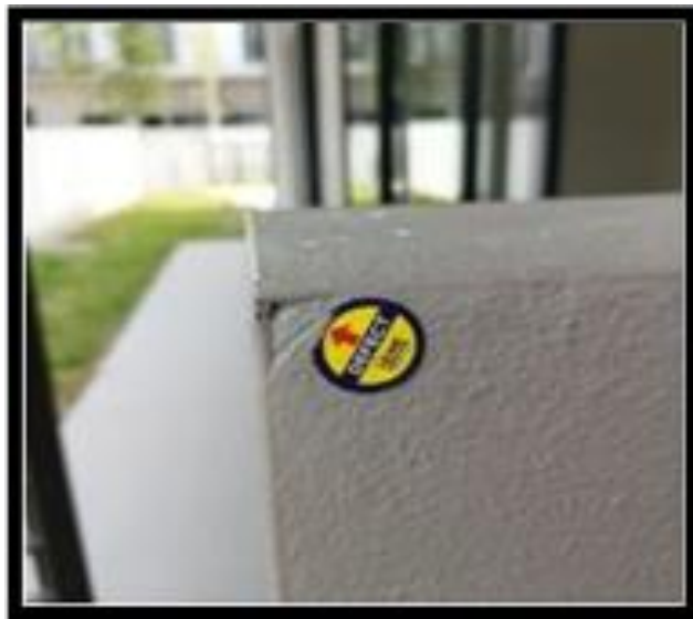
Figure 3.7: Chipping Wall.
