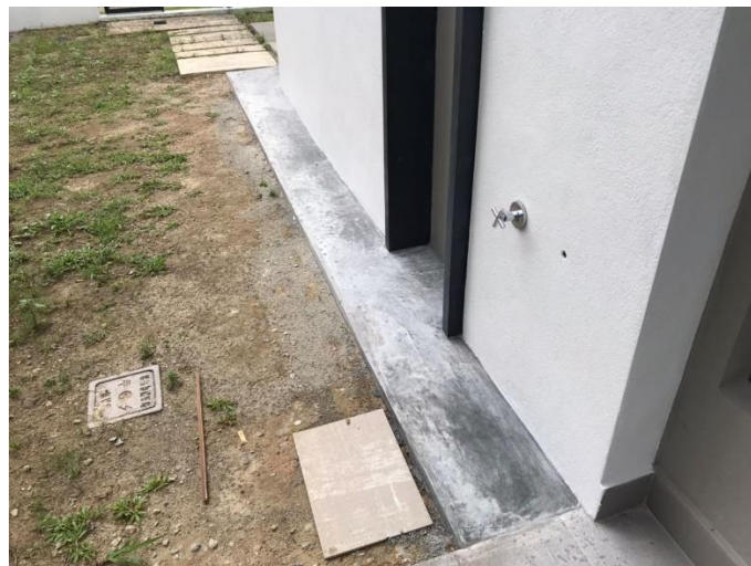
Figure 3.21: The Finished Work.
