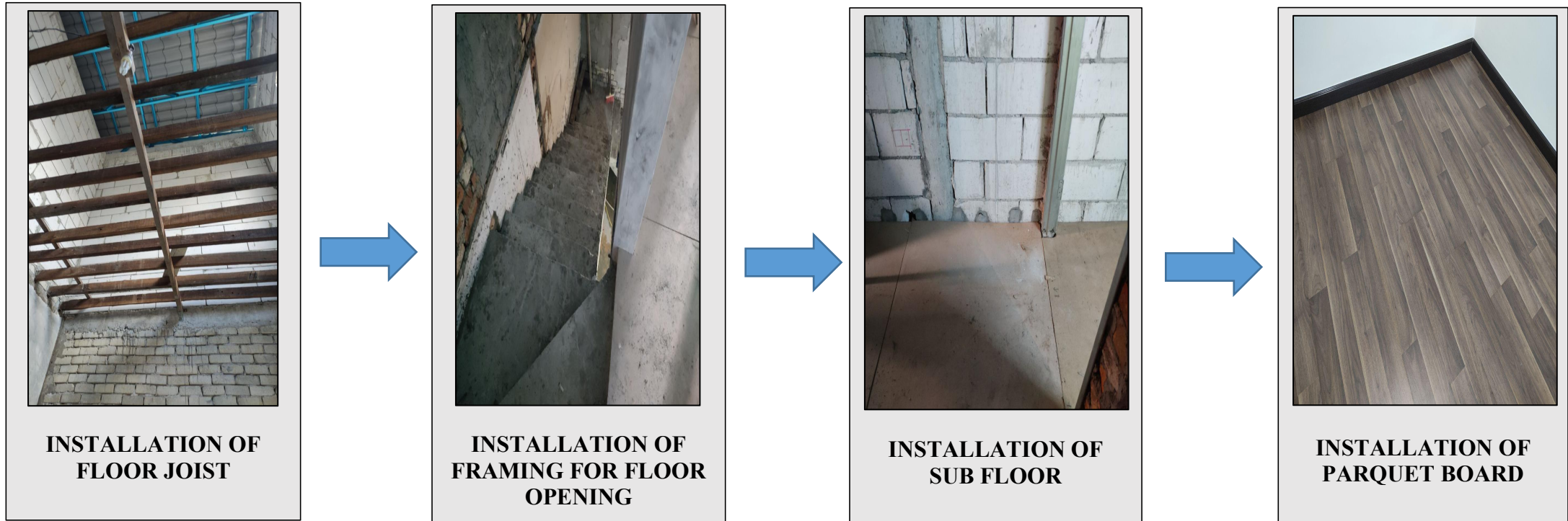
Figure 3.8: The diagram of parquet board installation
