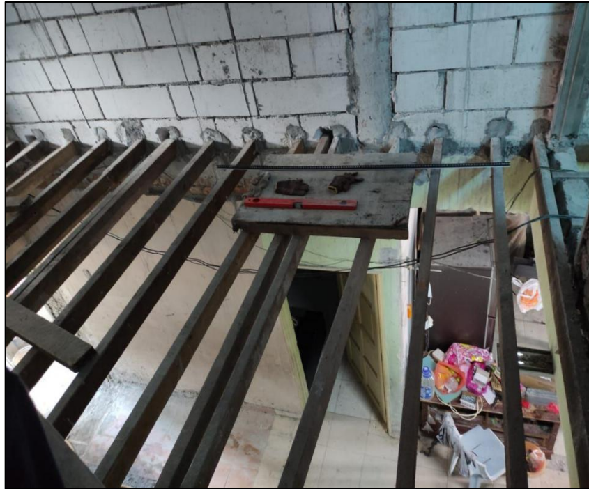
Figure 3.10: Top view of floor joist
