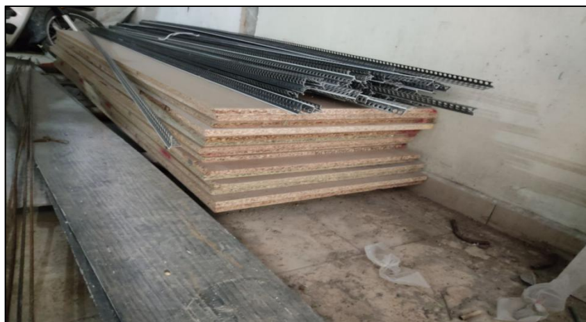
Figure 3.2: Plywood that are used for this project is store inside house.
