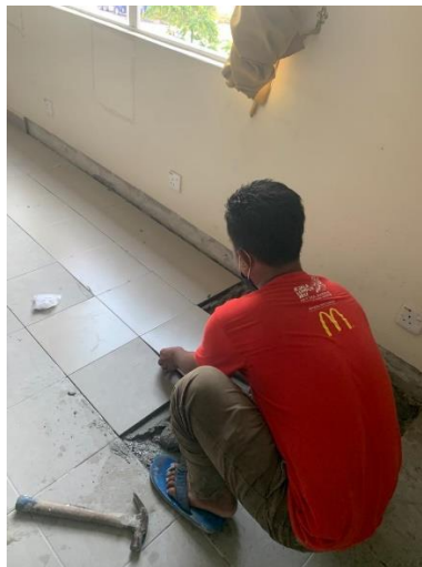
Figure 3.2h installation new tiles
