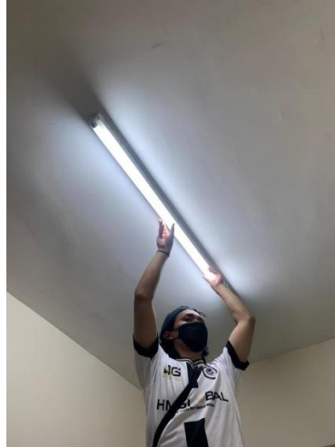
Figure 3.2d replaces new the fluorescent light
