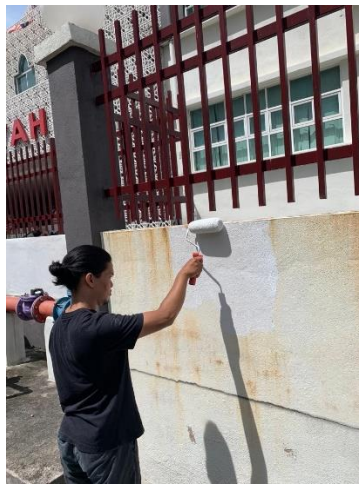
Figure 3.2g painting work to enhance building looks
