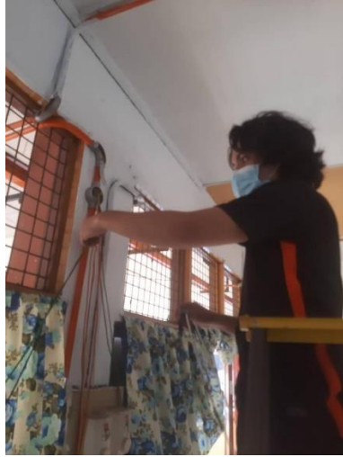
Figure 3.2f installation of wire
