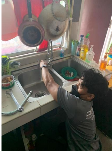
Figure 3.2i installation new water faucet
