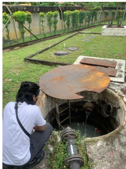
Figure 3.2b checking and inspection sewage treatment plant
