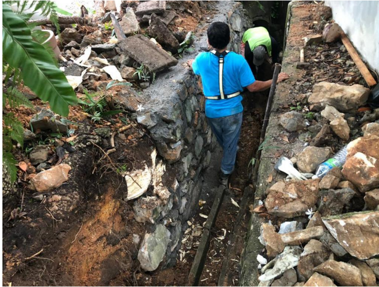
Figure 3.5: Breaking the damaged parts
