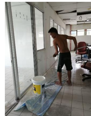
Figure 11: Application of undecoat paint on wall
