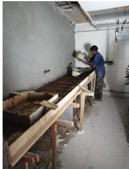
Figure 6: Construction of concrete bench
