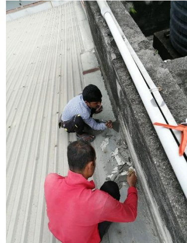
Figure 7: Removal of existing silicone
