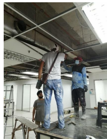
Figure 12: Labourers removing existing a/c ducts
