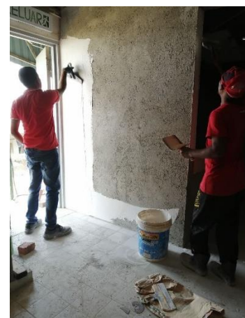
Figure 8: Application of skim coat on wall
