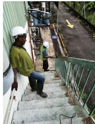
Figure 9: Labourers painting on staircase
