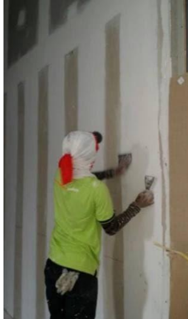
Figure 3.2.2.12: Plastering the wall
