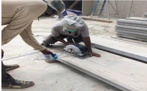
Figure 3.2.2.5: Cutting the panel
