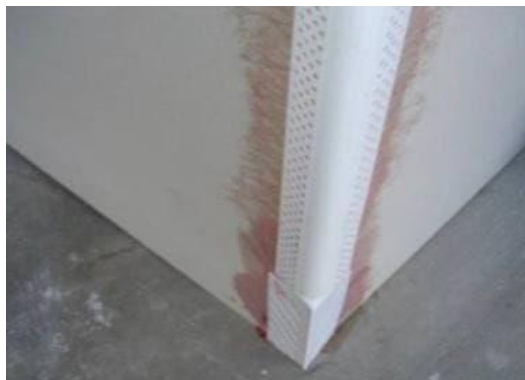
Figure 3.2.2.13: Install the corner bead
