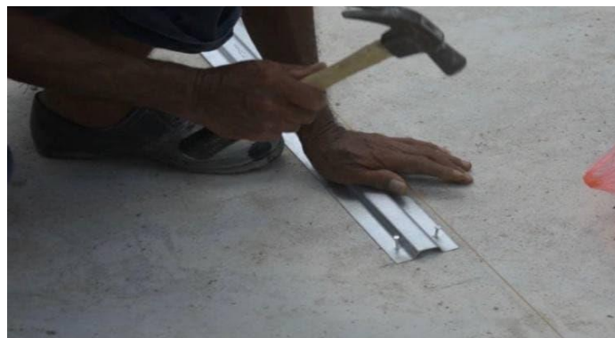
Figure 3.2.2.2: Installation of bottom track
