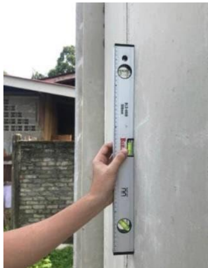
Figure 3.2.2.6: Measure panel straightness
