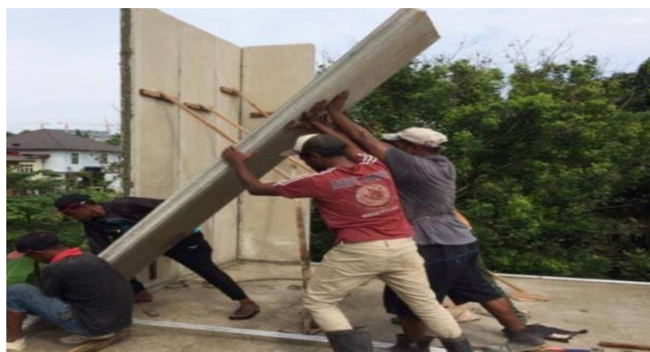
Figure 3.2.2.4: Installation of panel
