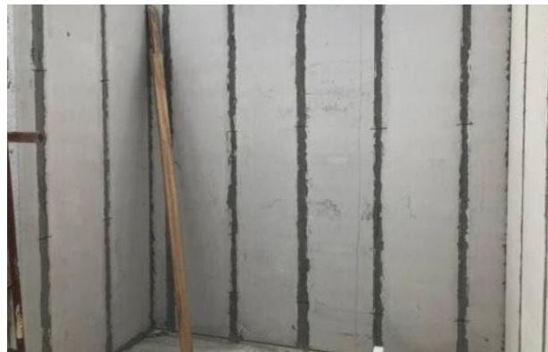
Figure 3.2.2.11: Applying mortar cement
