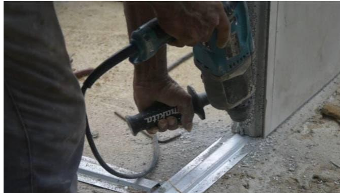
Figure 3.2.2.7: Hacking the panel
