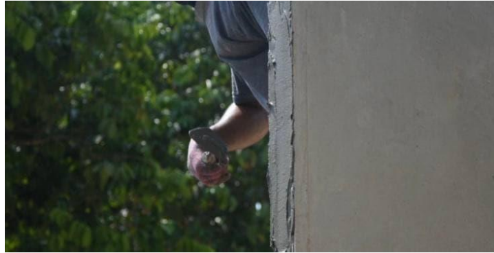
Figure 3.2.2.3: Applying Sika Ceram 288
