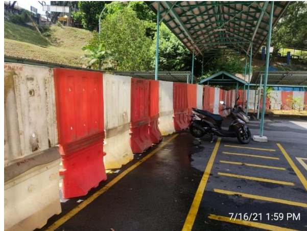
Site covered by barrier (figure 3.1.2)
