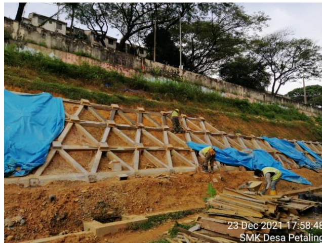
Figure 3.2.10.1 construct nail head
