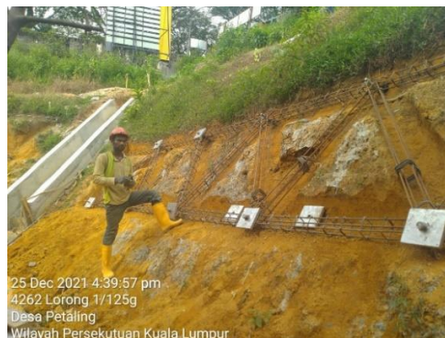
figure 3.2.7.2 install steel plate
