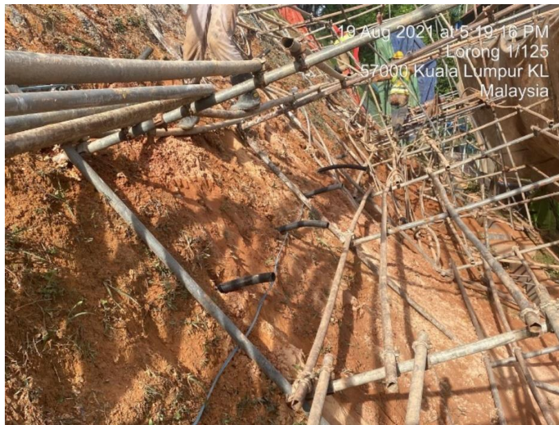
Figure 3.2.4.1 steel bar who has been installed
