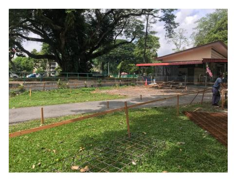
Figure 3.1 Contractor marks the area to be excavate
