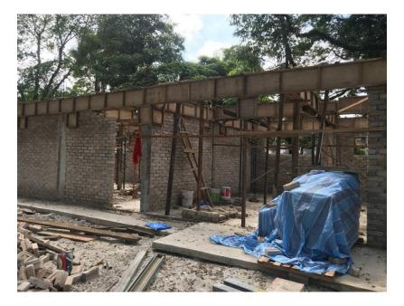
Figure 3.4 Beam has been installed
