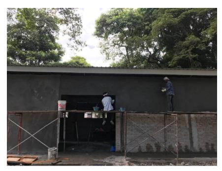
Figure 3.5 The contractor plaster the wall
