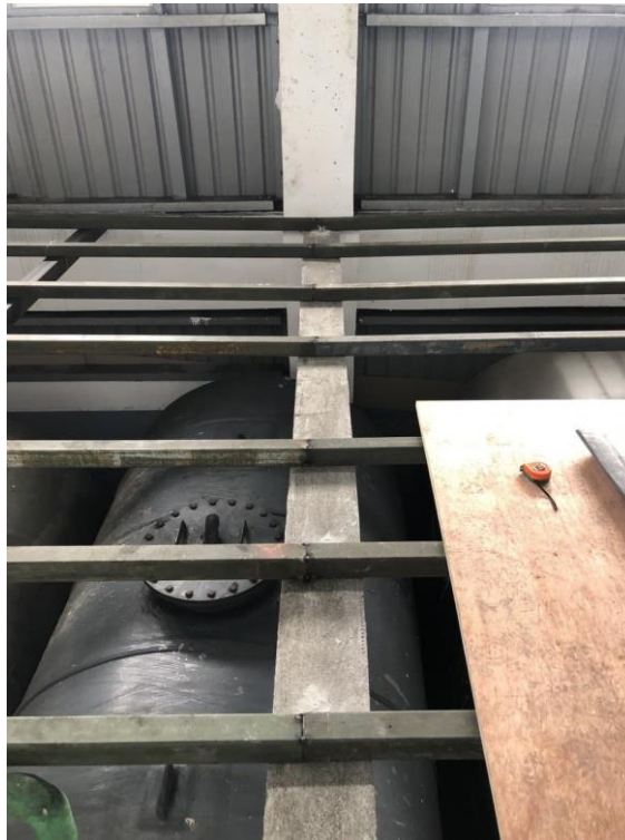
Figure 3.11 shown the hollow steel that been welded
