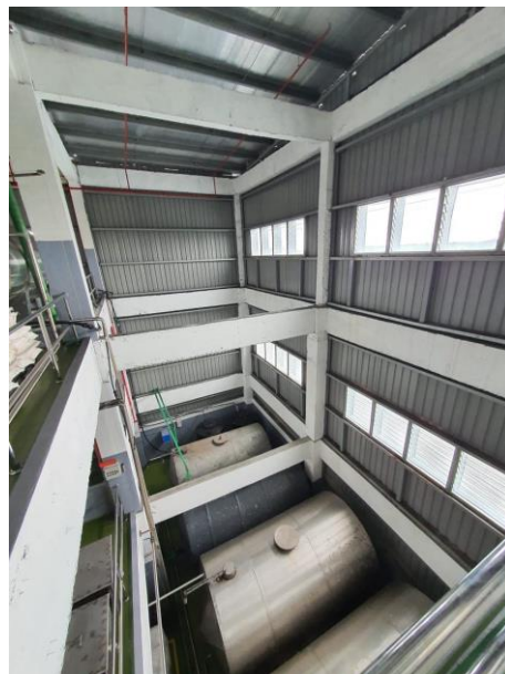
Figure 3.3 shown the area that need temporary structures
