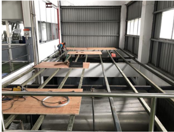
Figure 3.10 shown the hollow steel temporary structure for the platform
