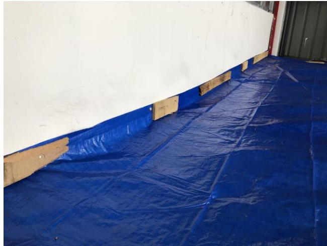
Figure 3.15 shown the canvas that been nailed to the wall
