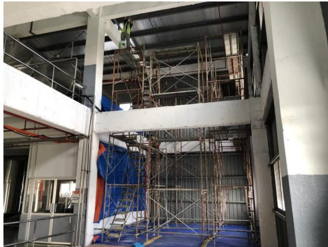
Figure 3.23 shown the complete temporary structure(scaffolding)
