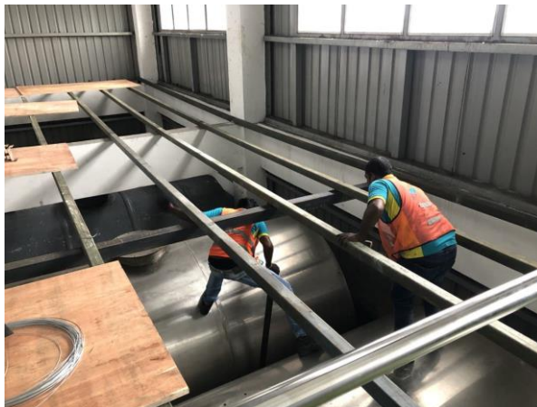
Figure 3.7 shown the labours setting up the hollow steel in position
