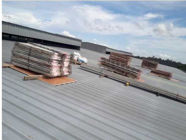
Figure 3.4 shown the component of scaffolding
