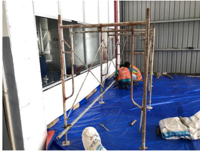
Figure 3.20 shown the labours clamp the scaffold tube to the frame
