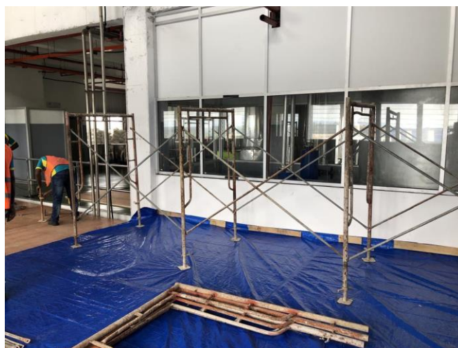
Figure 3.19 shown labours start setting up the scaffolding
