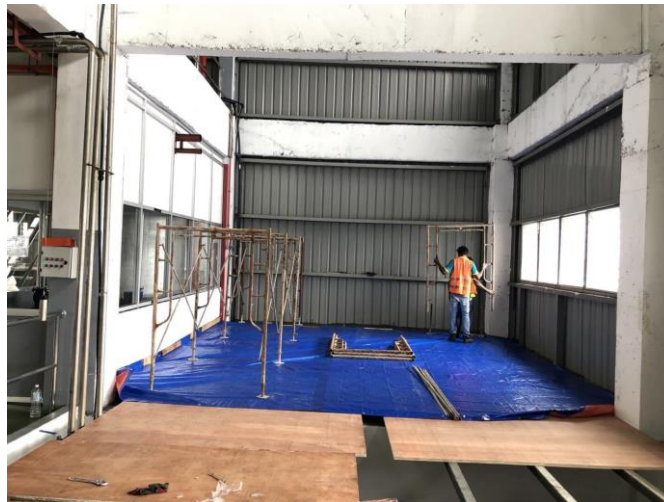
Figure 3.18 shown labours start setting up the scaffolding
