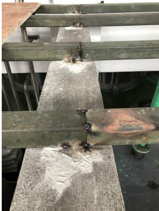
Figure 3.9 shown the hollow steel that been welded to the beam
