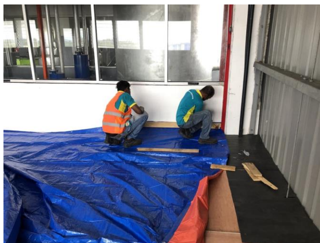
Figure 3.14 shown the labours nailing the canvas to the wall
