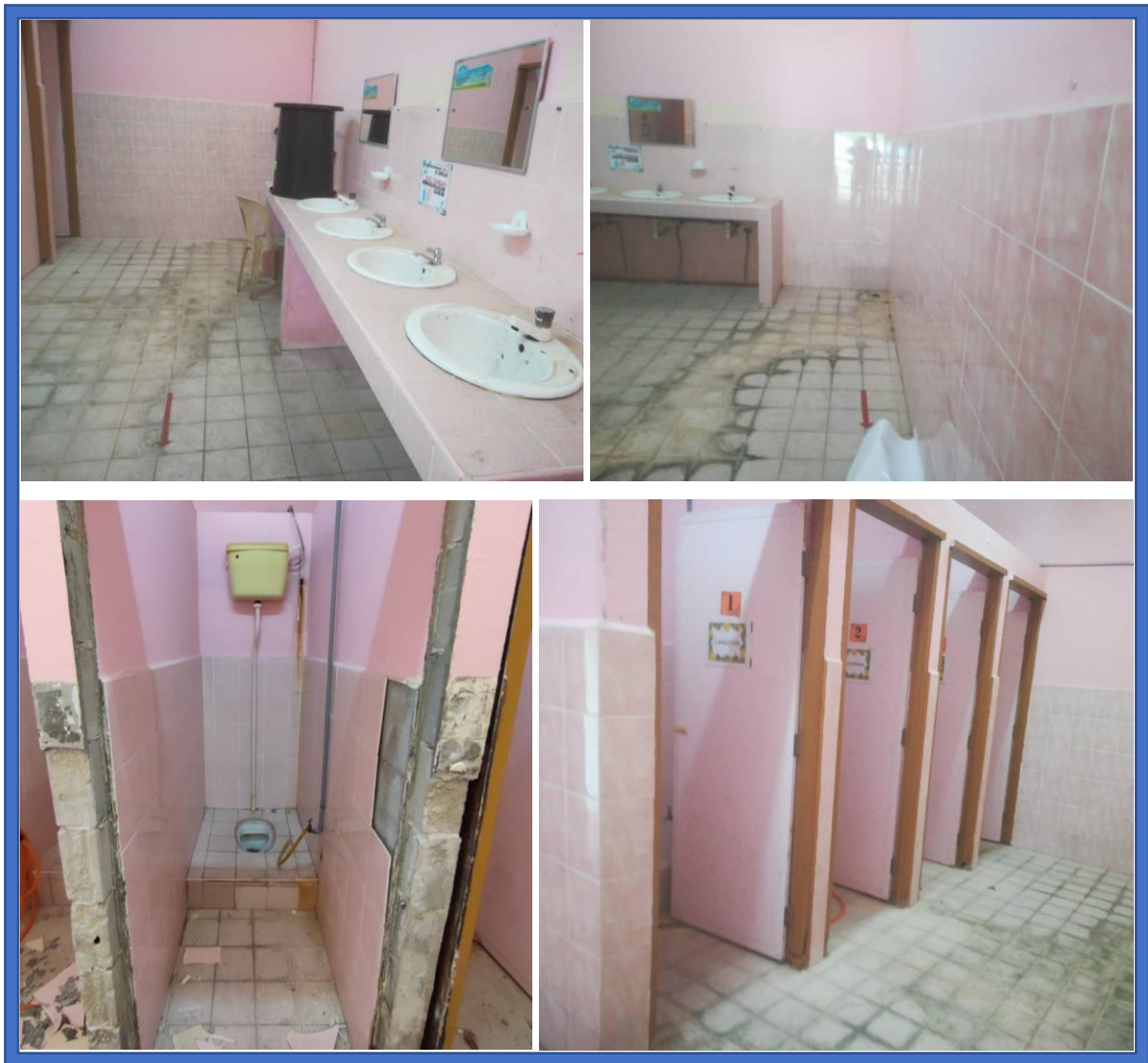
Figures 3.3.6.1: The toilet exterior during the project.
