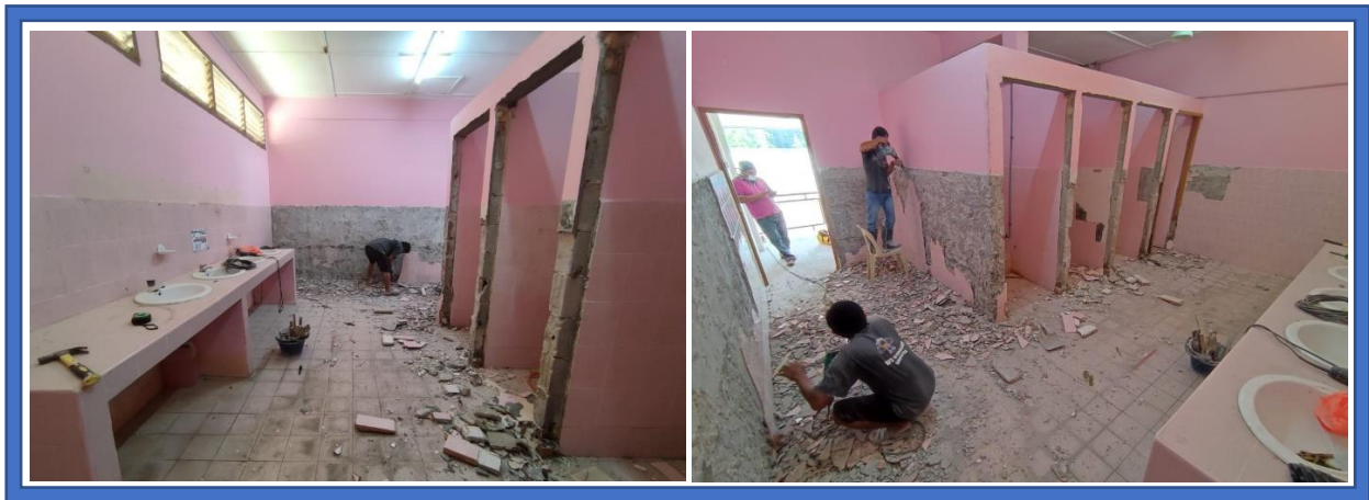
Figures 3.3.2.2: During the Site Preparation.
