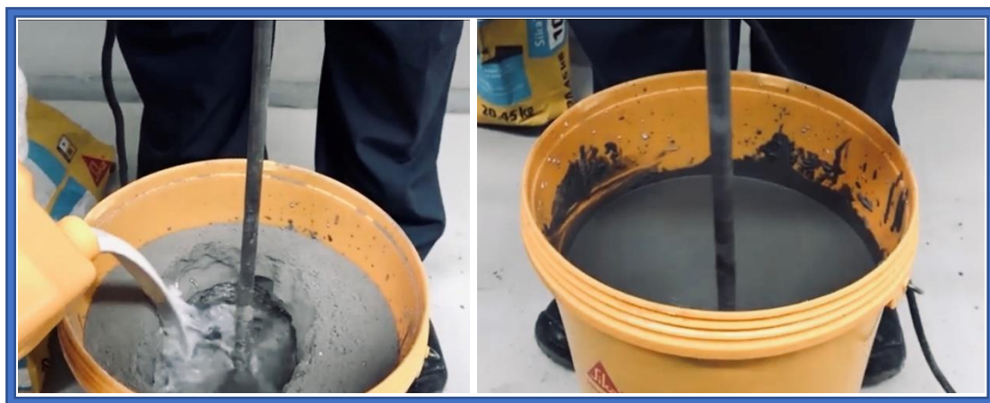
Figures 3.3.3.2: The mixing Process of the Cementitious Waterproofing Slurry.
