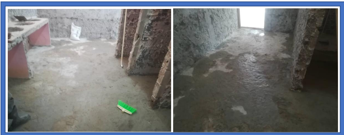
Figures 3.3.2.3: After the Site Preparation.
