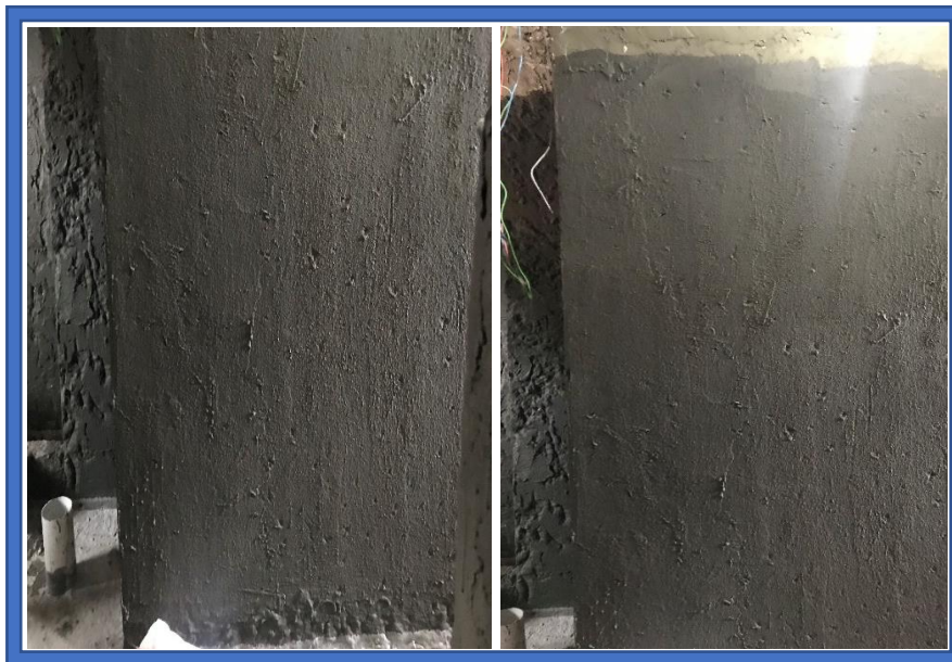
Figures 3.3.3.4: After the Cementitious Waterproofing Slurry are applied on the wall.
