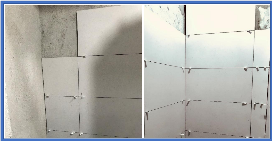
Figures 3.3.4.2: During the tile's installation.
