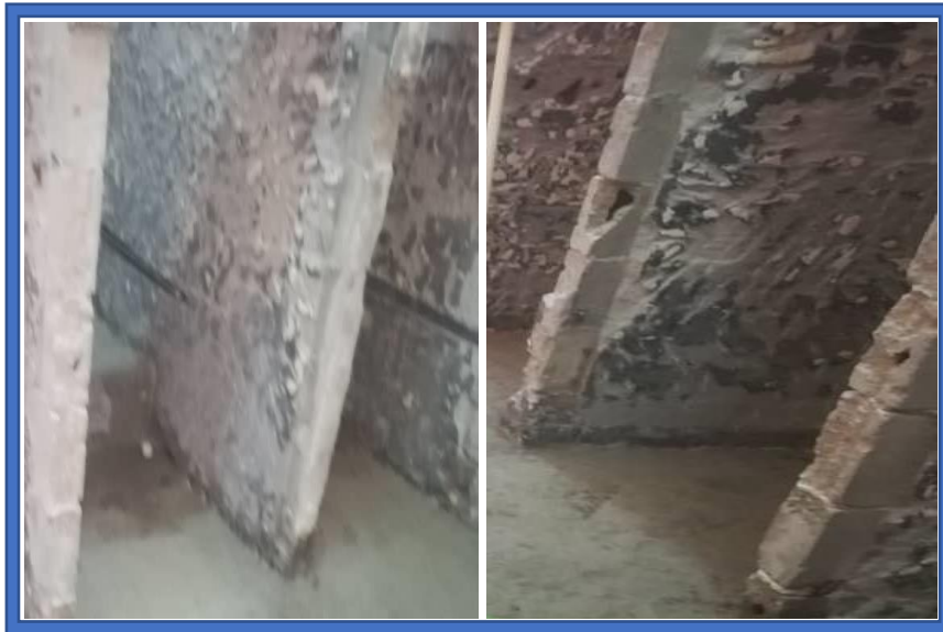
Figures 3.3.3.4: Before the Cementitious Waterproofing Slurry are applied on the wall.
