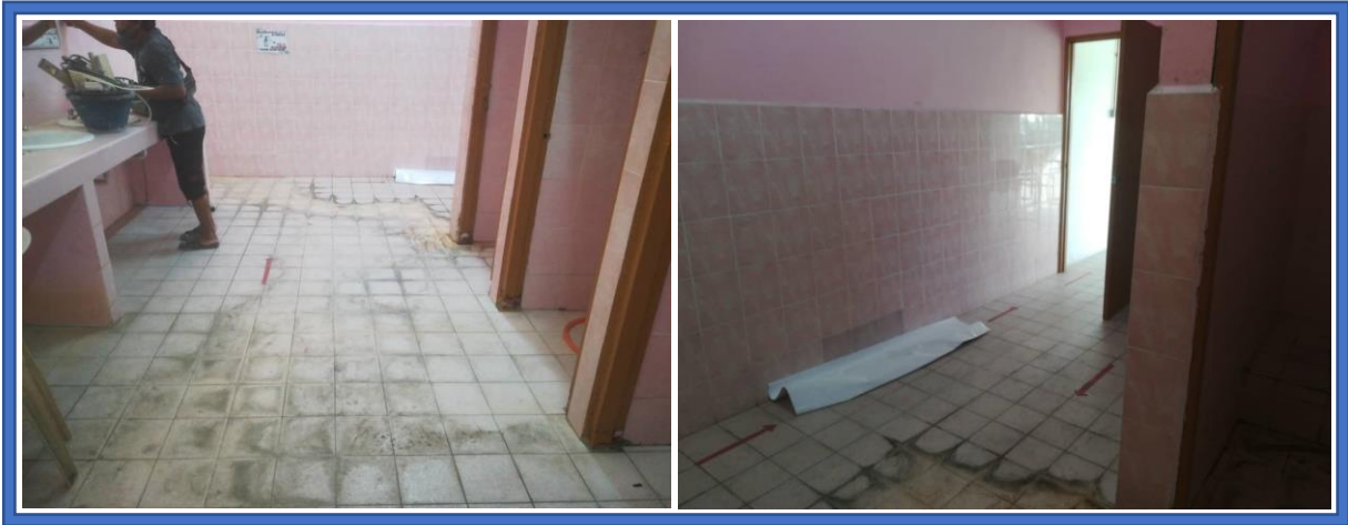
Figures 3.3.2.1: Before the Site Preparation.
