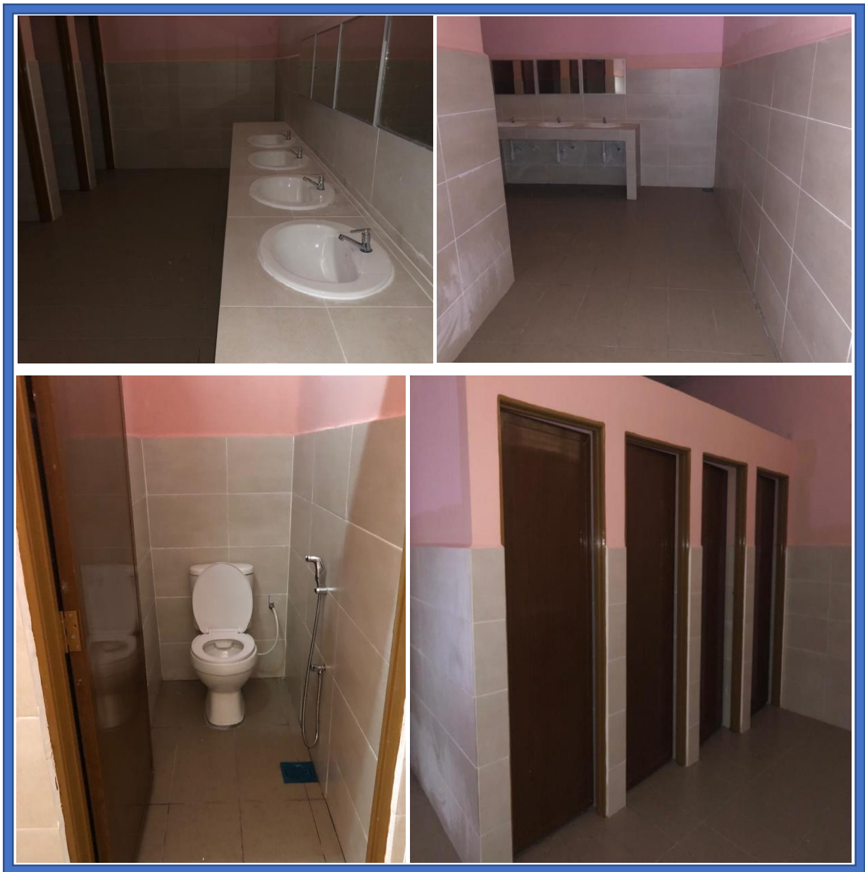
Figures 3.3.6.2: The toilet exterior after the project.
