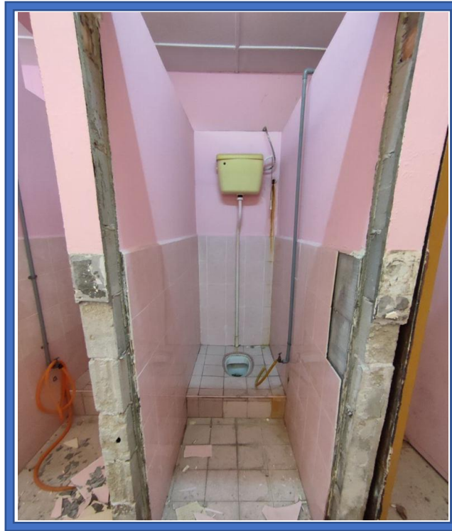
Figures 3.3.5.1: Before the fixtures are installed.
