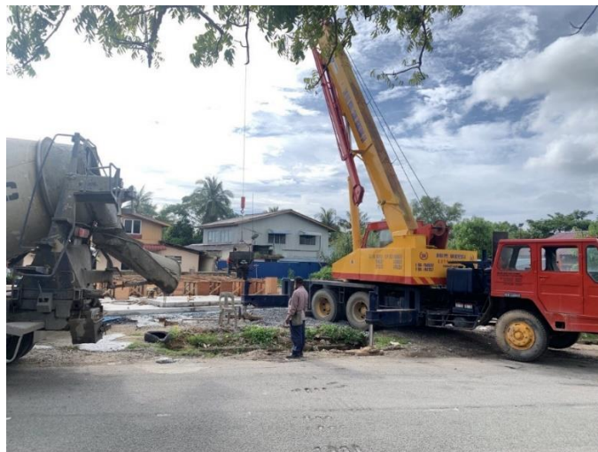
Figure 11: Pouring concrete using crane
