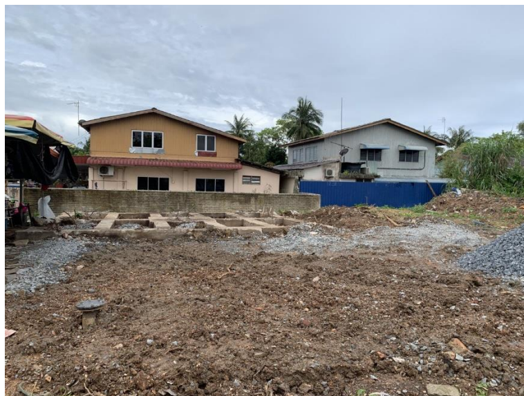
Figure 4: View of pump house construction site from infront
