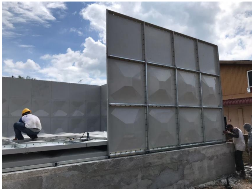
Figure 17: Proses of installing HDG
