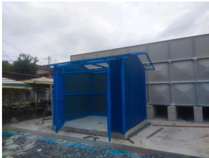
Figure 15: Almost completed Pump House
