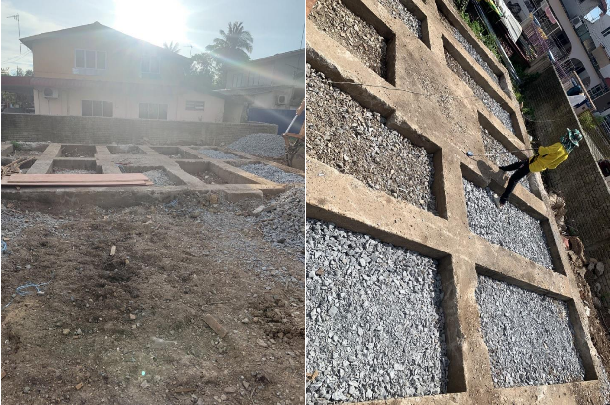
Figure 6: Backhoe loader pouring crusher run in slab area
