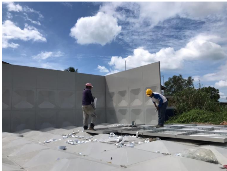
Figure 13: Installing FRP Water Tank
