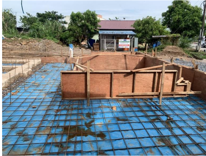
Figure 10: Pump house formwork
