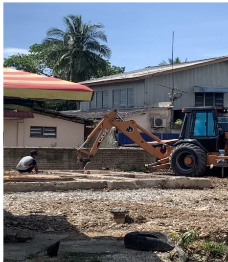
Figure 5: Backhoe loader digging and pouring soil in slab area
