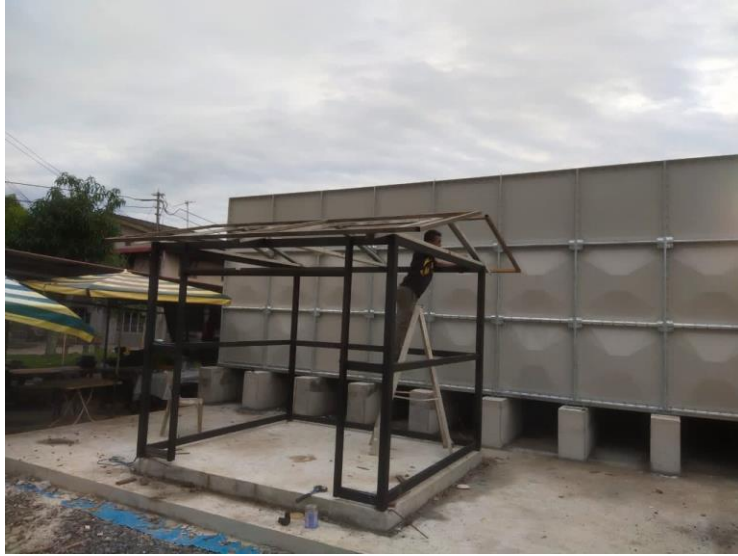
Figure 14: Pump House Structure
