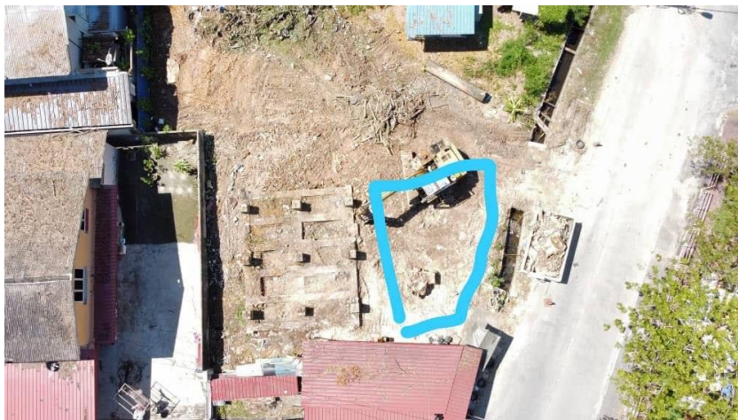
Figure 1: View of the site taken from drone
