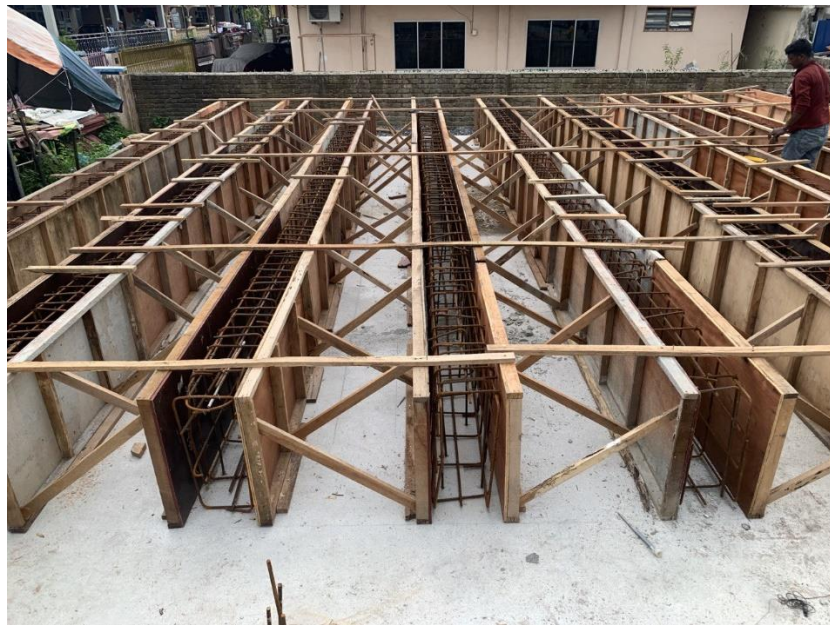
Figure 9: Formwork and plinth beam
