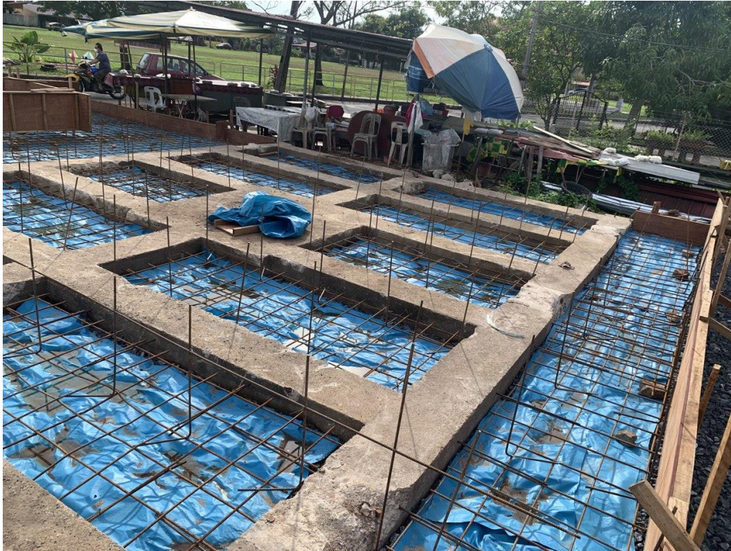
Figure 7: BRC Steel for slab
