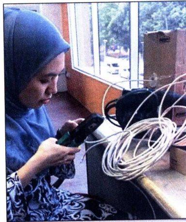
Figure 3.14 Installing Ethernet Cable
