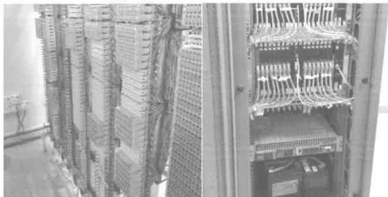
Figure 15: Communication Unit Site Visit
