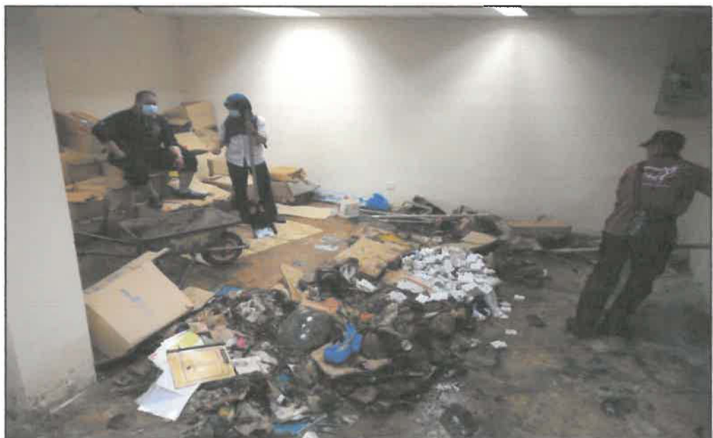
Figure 3.26: The damaged records found
