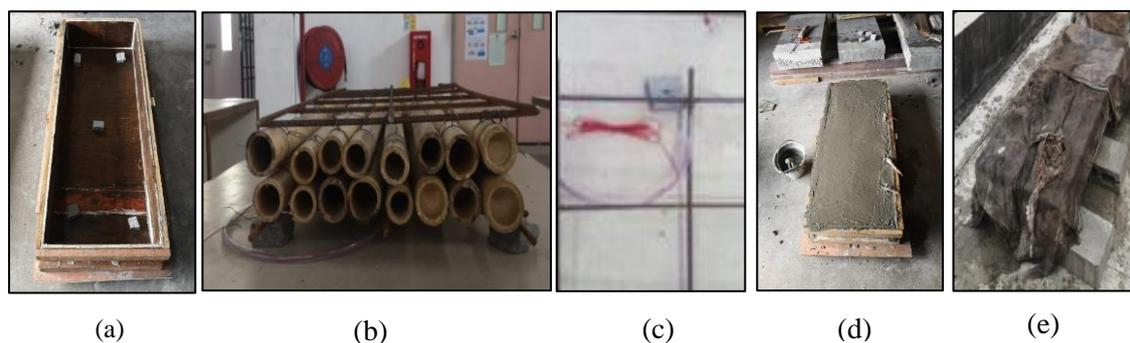
Figure 4: Casting of the slab (a) Formwork of Slab; (b) Arrangement Sandwich Between Mesh Wire and Bamboo; (c) Installation of Strain Gauge for BRC A8; (d) Slab concrete is completely levelled; (e) Wet Covering for Curing Process.
