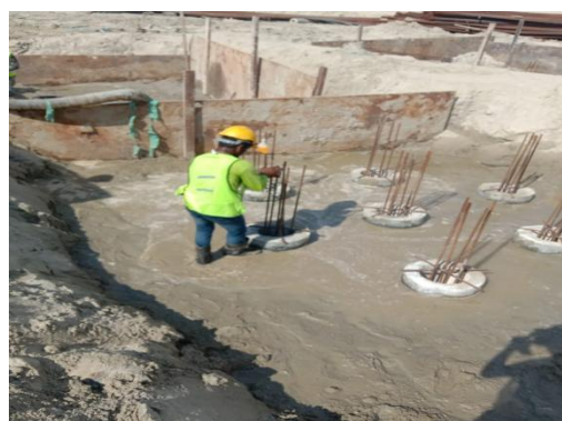
Figure 3.3.2: Pile Plug installation
