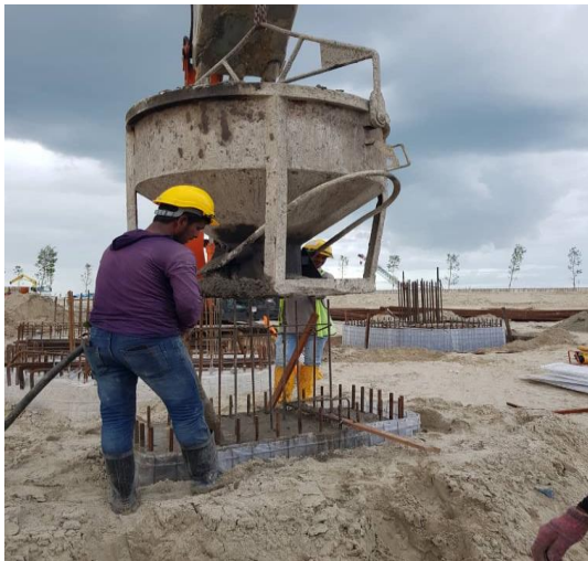
Figure 3.3.6: Concreting Pilecap
