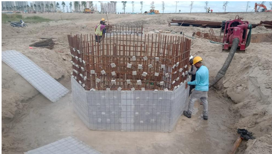
Figure 3.3.5: Installation of pecaform to pilecap rebar
