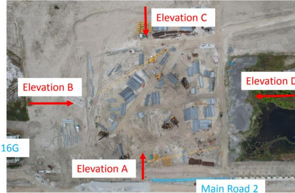
Figure 3.1.3: Overview of Construction Site.
