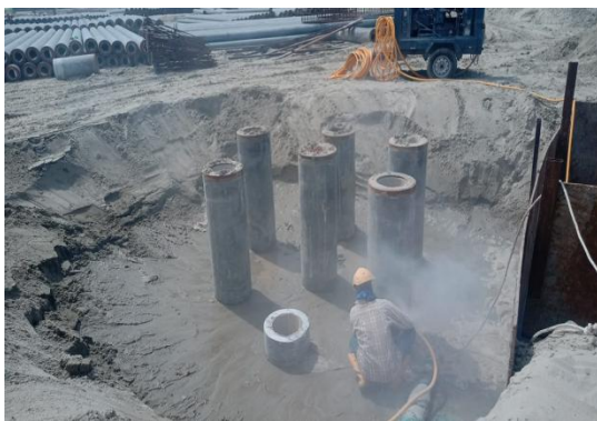
Figure 3.3.1: Cut-off Level Piling
