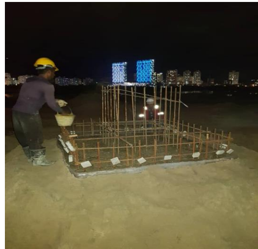
Figure 3.3.7: Finish Concreting pilecap work
