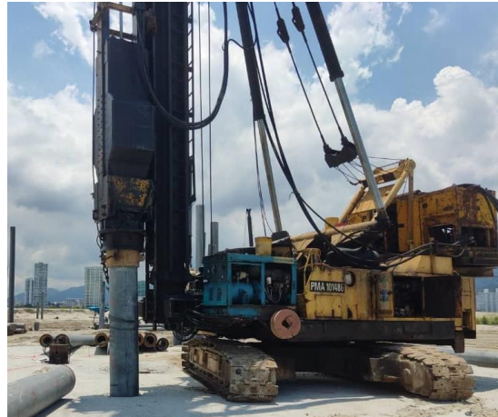
Figure 3.2.2: Driven pile
