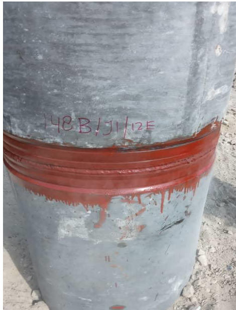
Figure 3.2.4: Joint of piling
