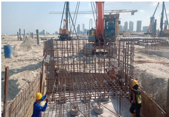
Figure 3.3.3: Installation of pilecap rebar
