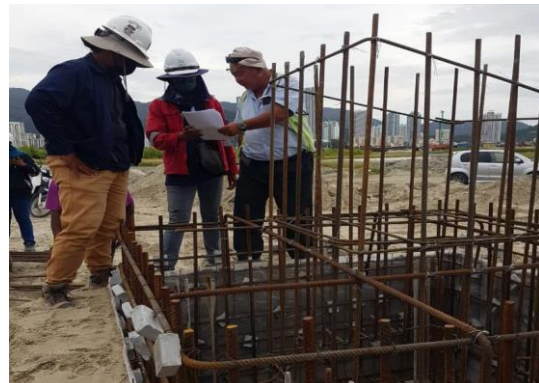
Figure 3.3.4: Inspection rebar for pilecap
