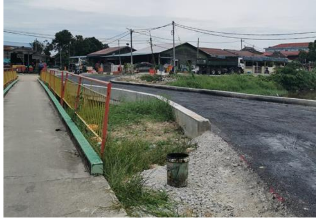
Figure 3.4: Applying the prime coat.
