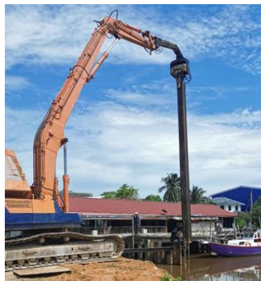
Figure 3.10: Vibrator hammer machine for driving steel sheet piles.
