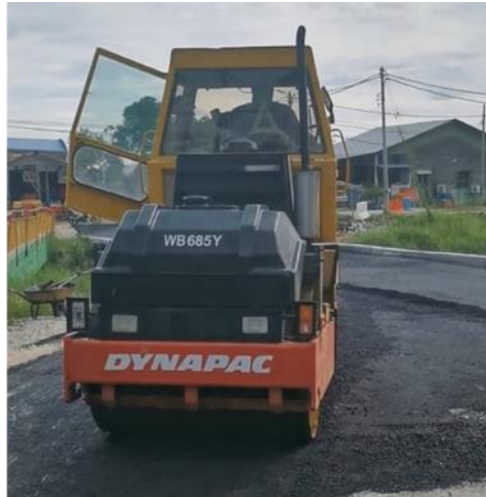
Figure 3.7: Road roller for compacting road surface.
