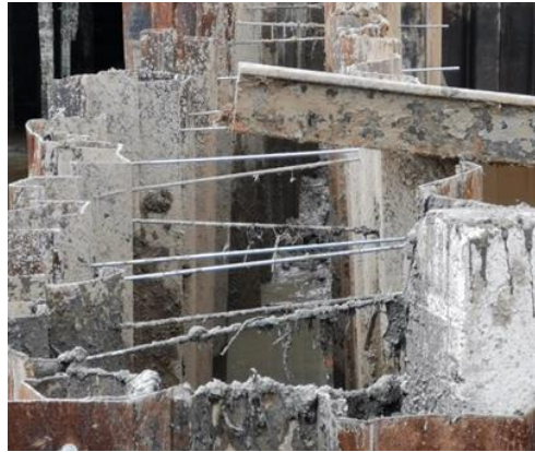
Figure 3.12: Braced sheet pile to undertaking deep excavation.
