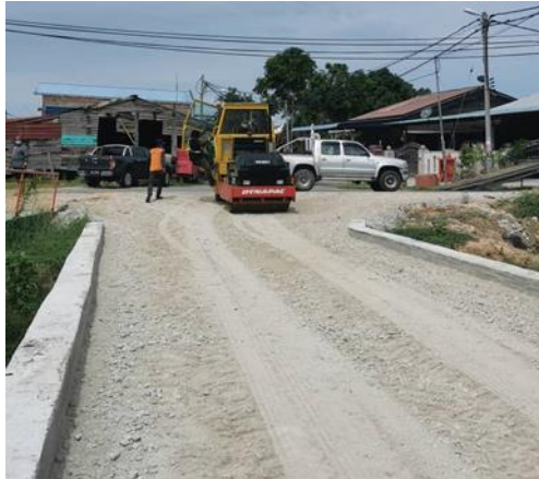
Figure 3.3: The road surface has been compacted.
