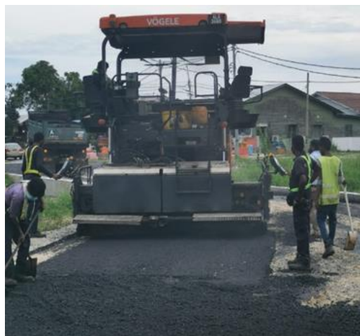
Figure 3.5: Using a premix coat of premix carpet.
